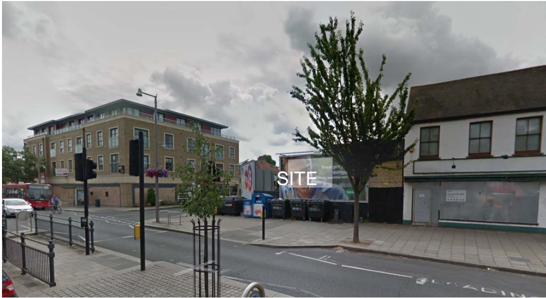
HEATH ROAD SHOWING BEAUMONT HOUSE AND EXISTING BUILDING ON SITE
