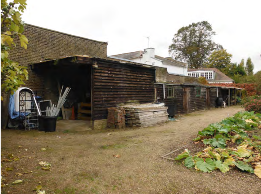
Photo 5 – Workshops/sheds in the SW site corner (looking SW)
