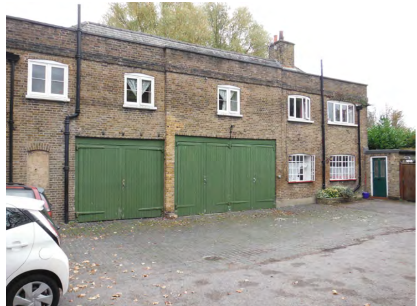
Photo 4 – Building in the SE corner of the site (looking SE)
