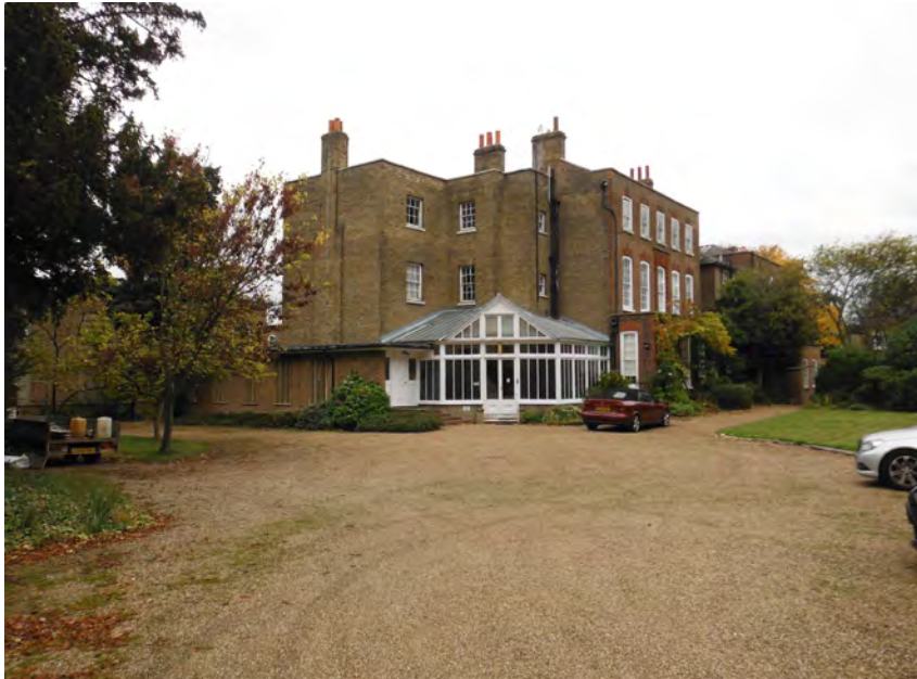
Photo 1 – View of existing building from the SW site corner (looking NE)
