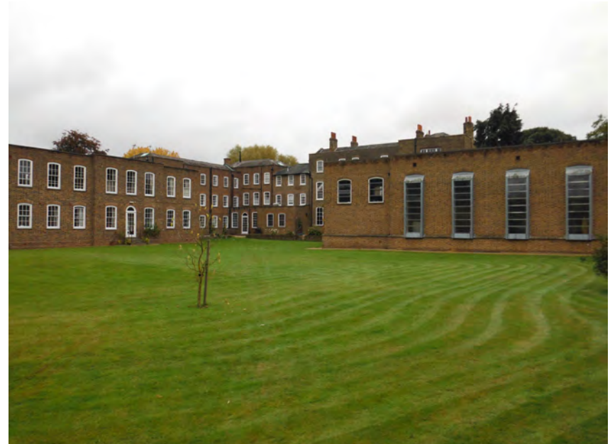
Photo 2 – View of existing building from site centre (looking SE)
