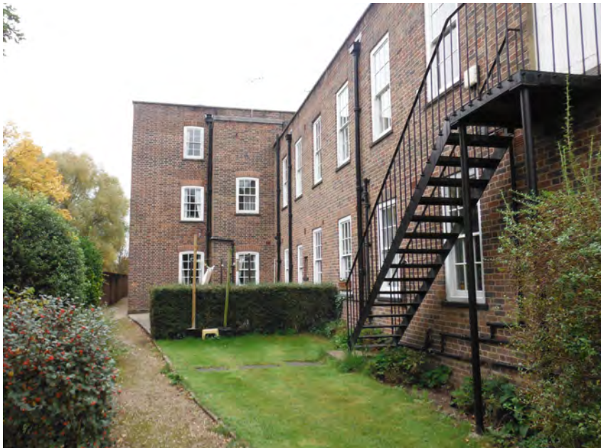
Photo 3 – View of eastern elevation of existing building (looking S)
