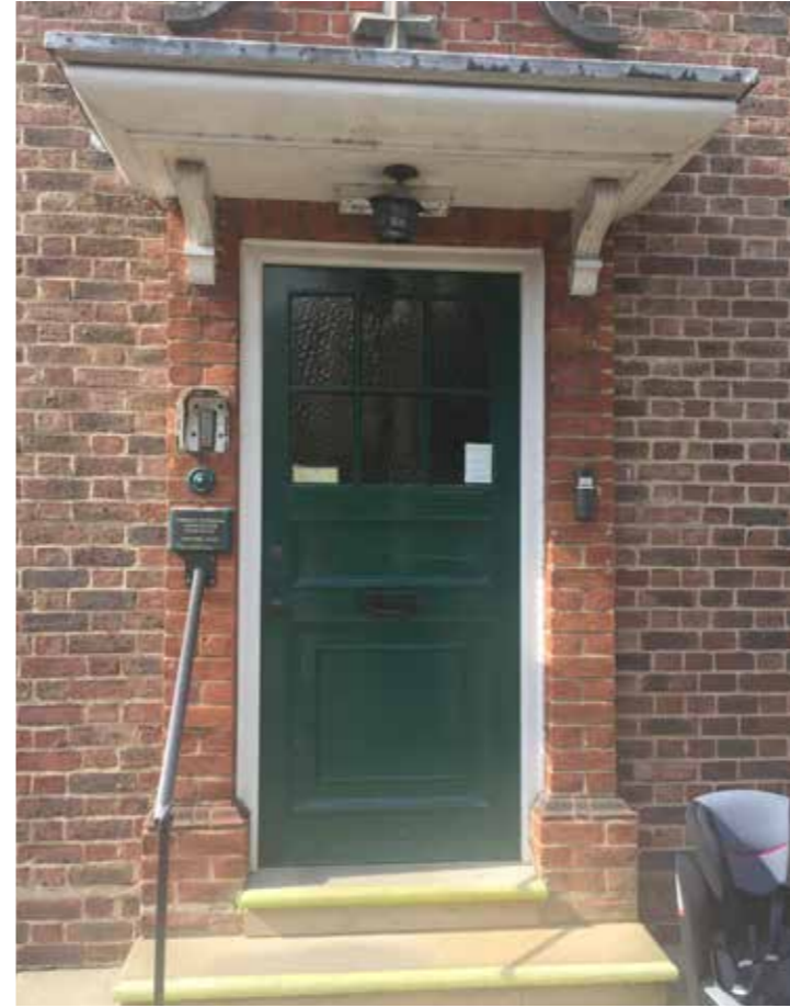
Main entrance to later wing (to be retained)
