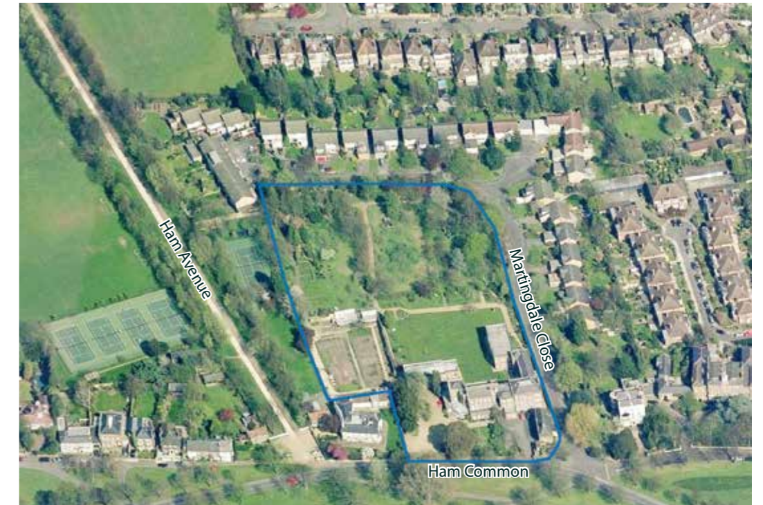
Aerial view of site looking north
