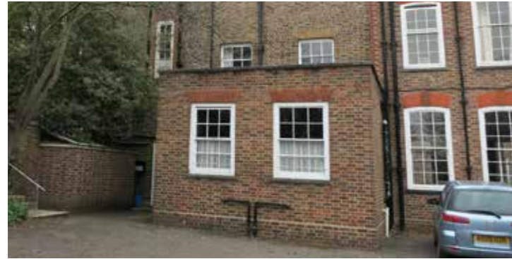
Front elevation later addition
