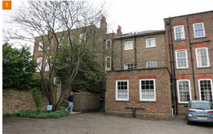
Listed building on site, South side
