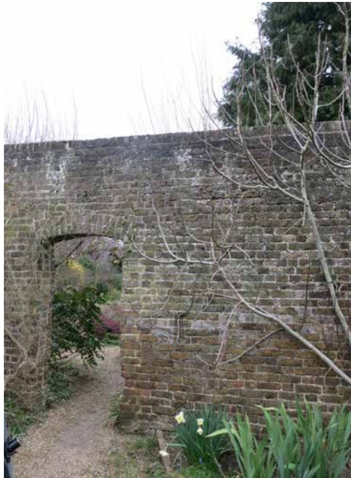
View of walled garden entrance
