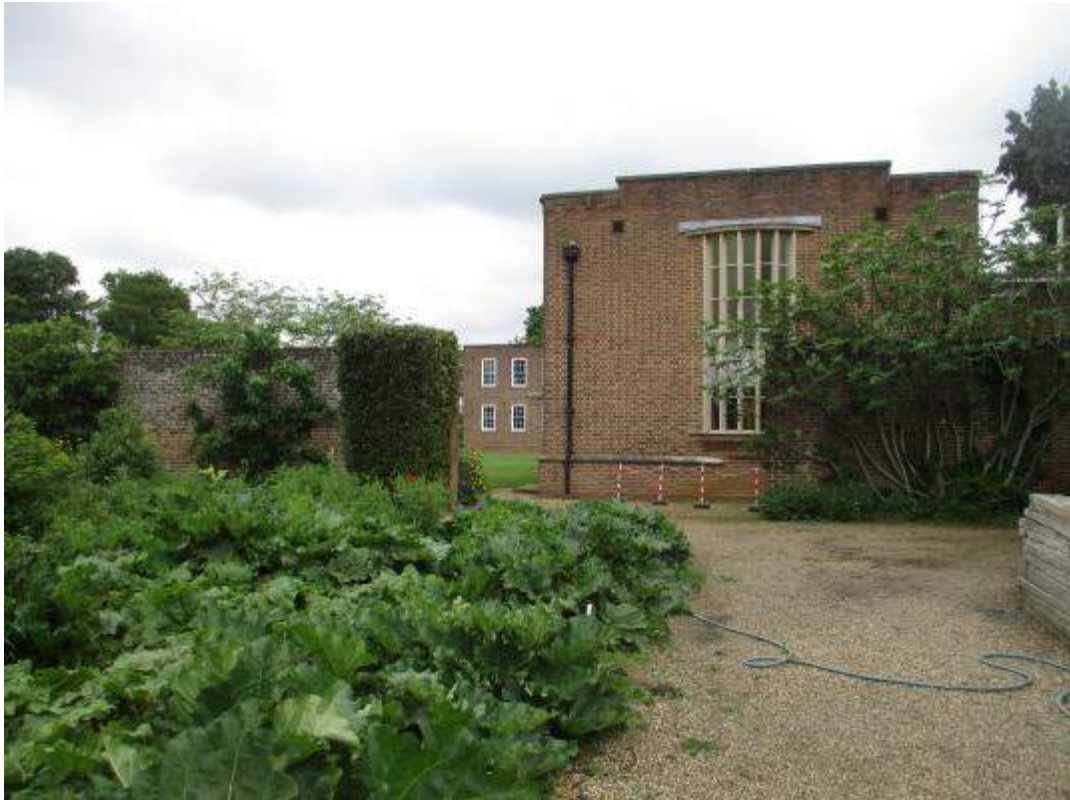
Photo 3: A view of the western façade, showing the modern extension
