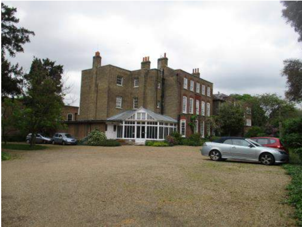
Photo 1: A view of the southern and western façade of St Michael's Convent
