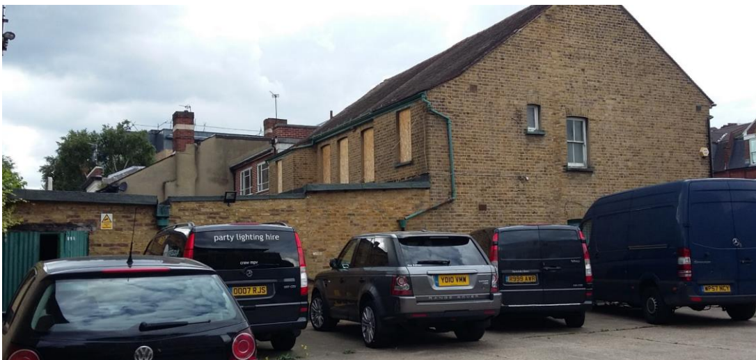
Photograph 2.1: Yard and side of building and single storey store
