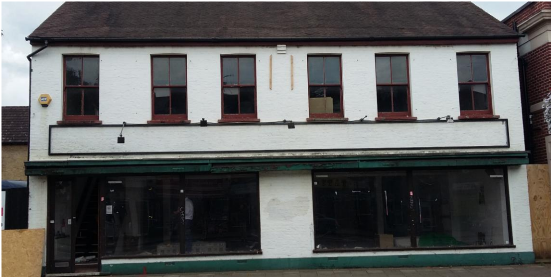
Photograph 2.3: Main building (149-151 Heath Road)
