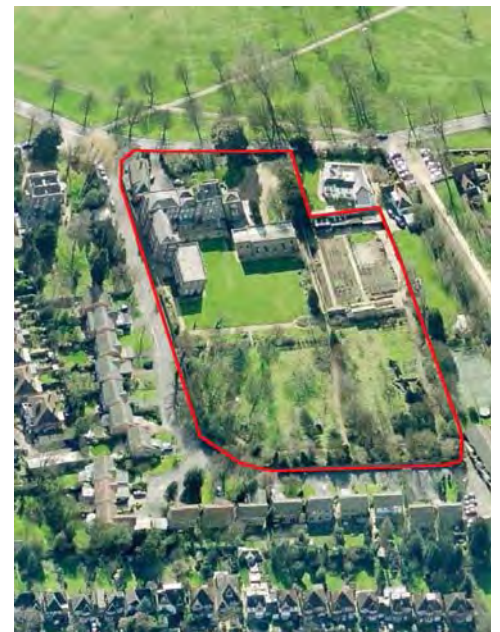
Aerial view of site looking south
