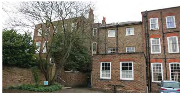
The front single storey extension
