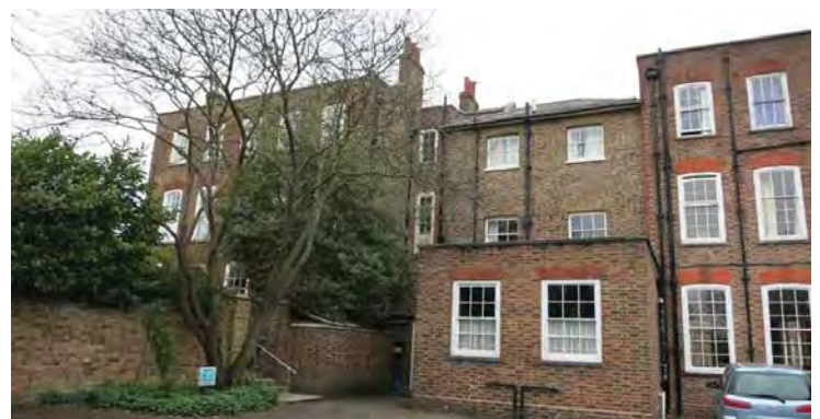
The front single storey extension
