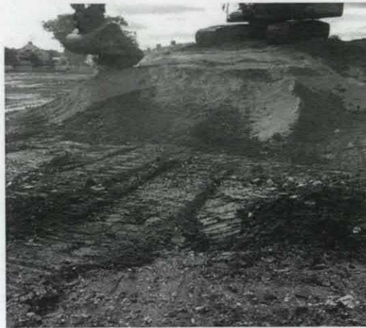
Stabilisation of stockpile 6
