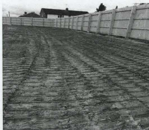
Natural ground after hotspot removal
