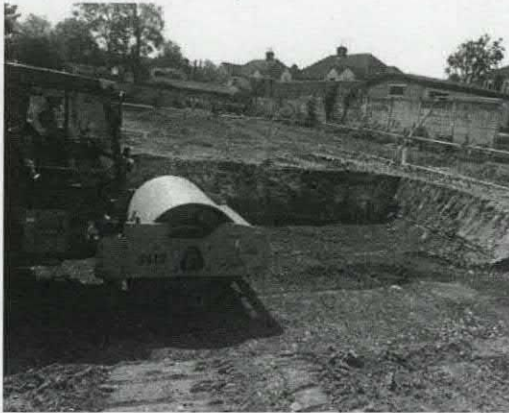
Compaction of stabilised material from stockpile 2 and 3
