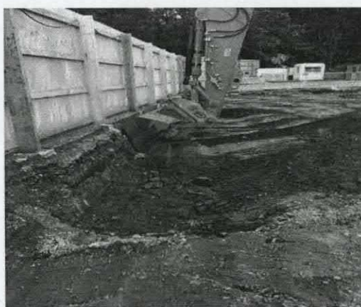
Excavation of Lead contaminated soils
