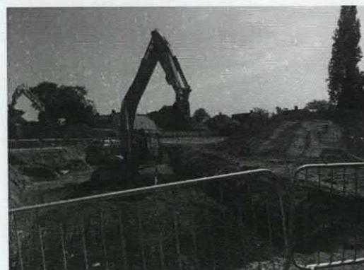
Placement of stabilised fill from SP2 and 3
