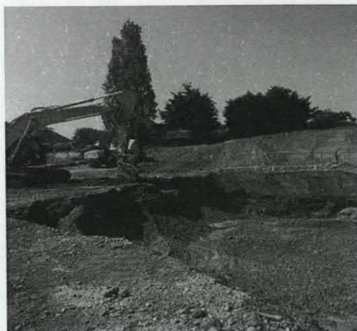
Excavation of road
