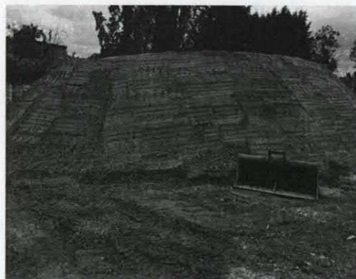
Remaining natural ground stockpiled
