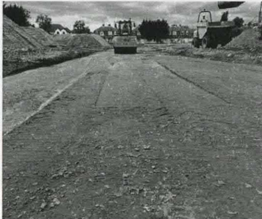
Compaction of natural stabilised clean cap
