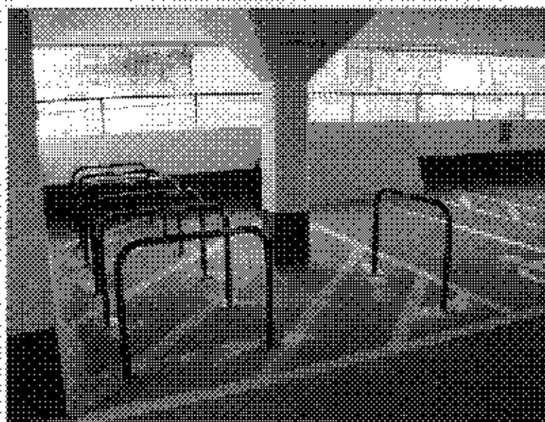
Figure 2.7 -Existing Cycle Stands Within a Car Park
