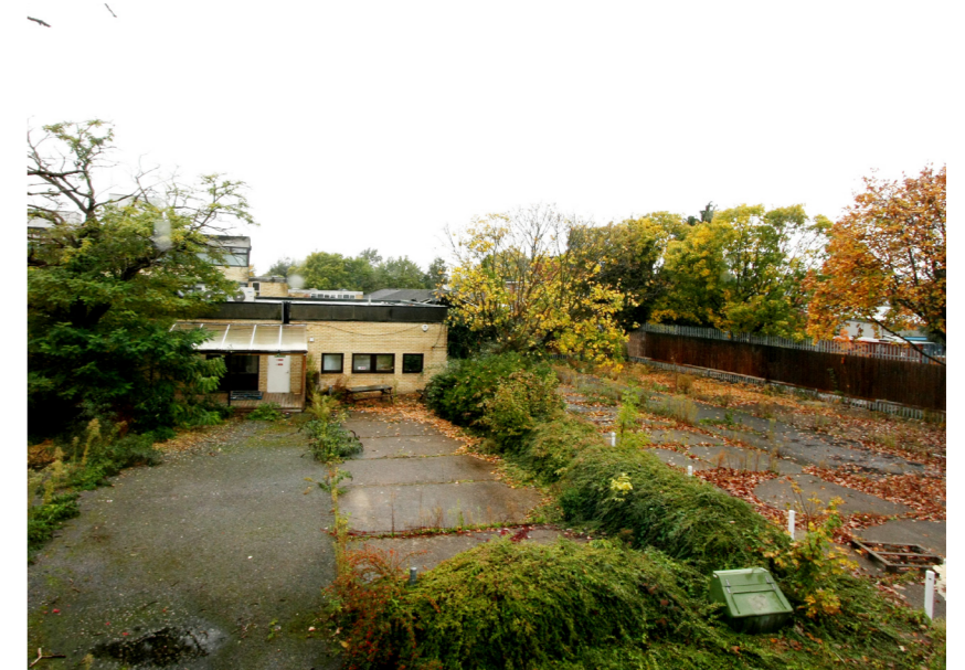
View looking Northwest to office building within site
