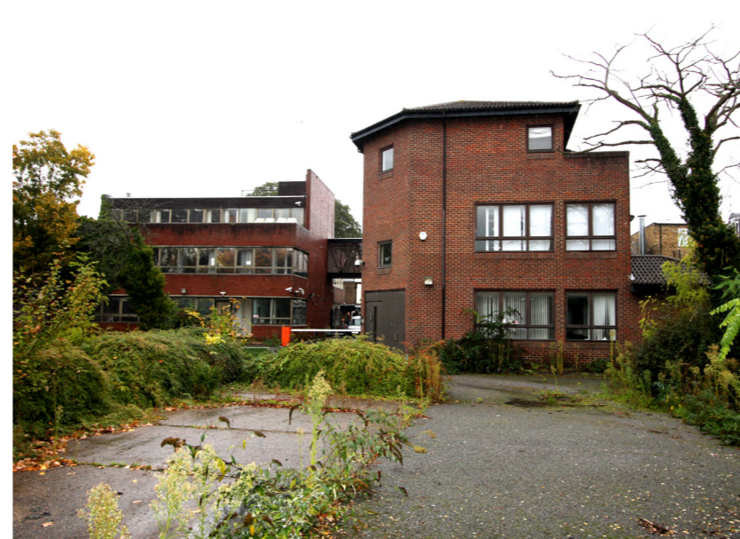
Northwest rear elevation 63-71 from within site Existing car park and hard-standing
