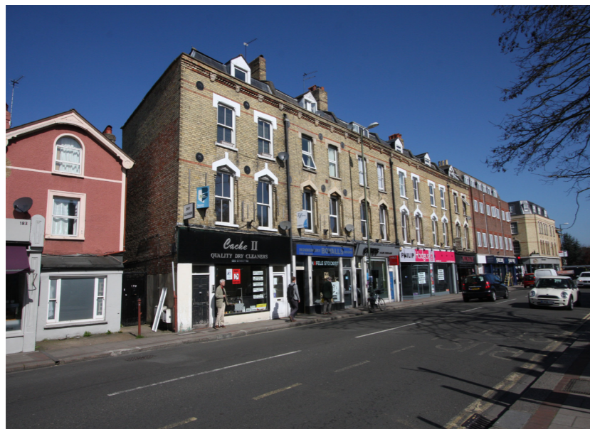
Tall 4 storey terraced buildings with mansard roofs
