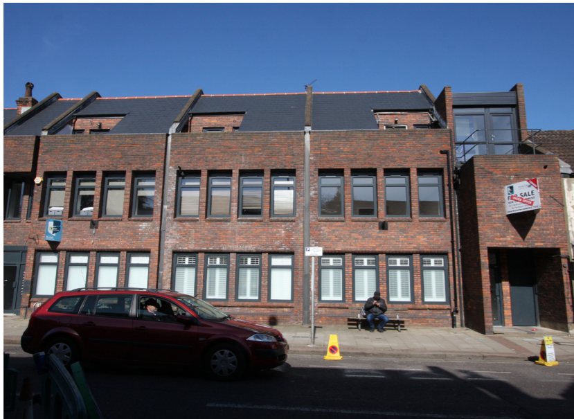
3 storey office converted to residential
