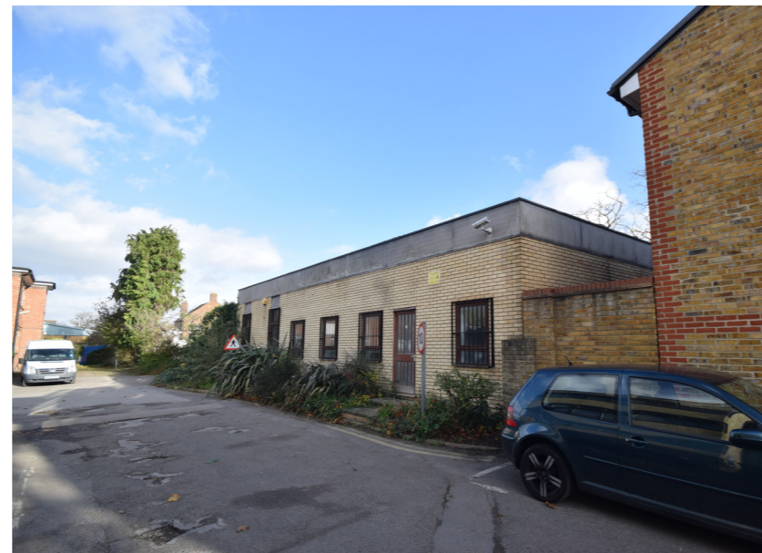
Office building located in northwest corner of the Site View from private access road
