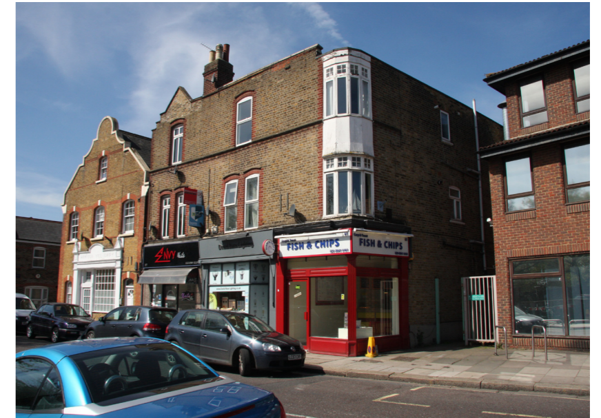
55-61 High Street looking South
