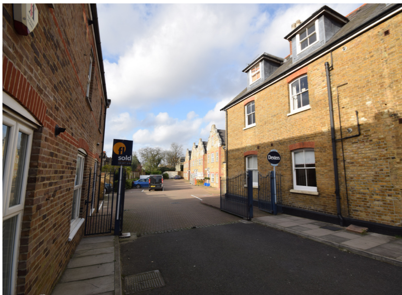
Side elevation to no.55 and access to rear Mews
