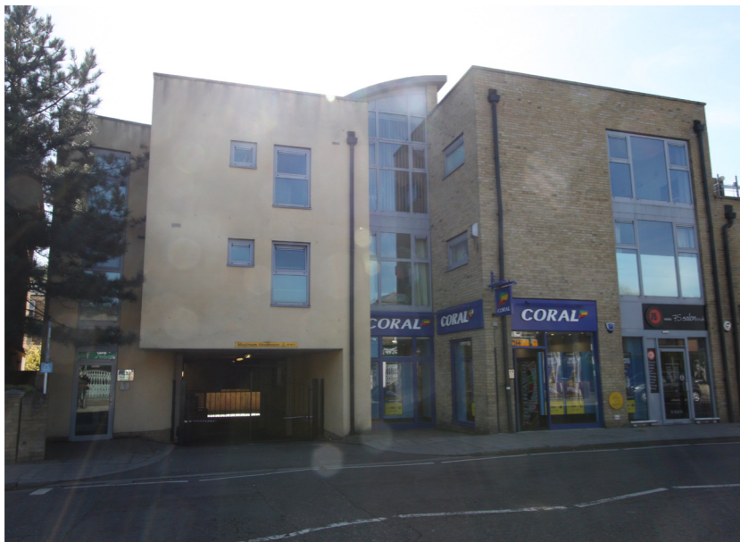
Tall 3+ storey mixed use development
