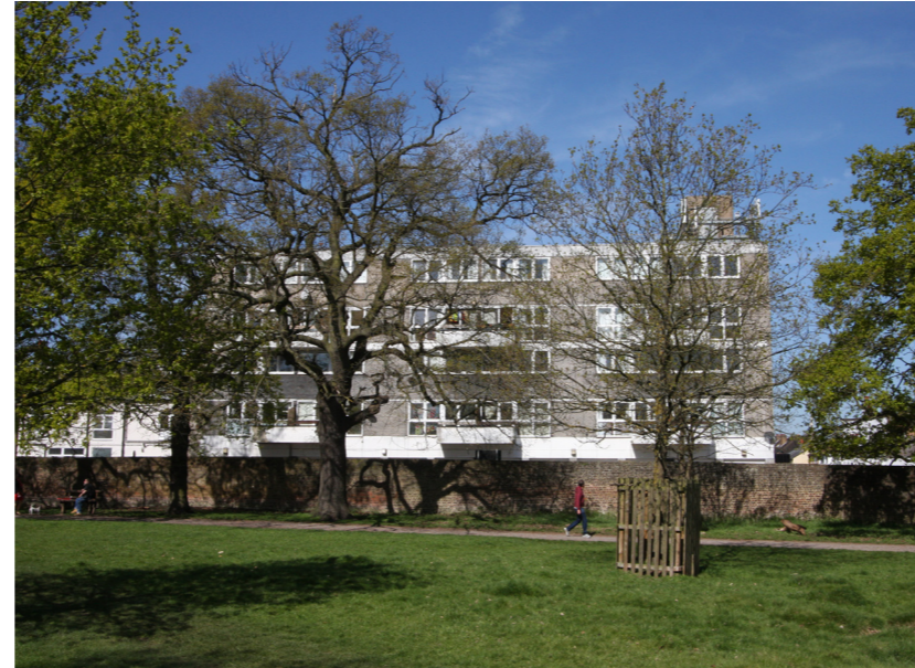
The Pavilion 5 storey flatted development
