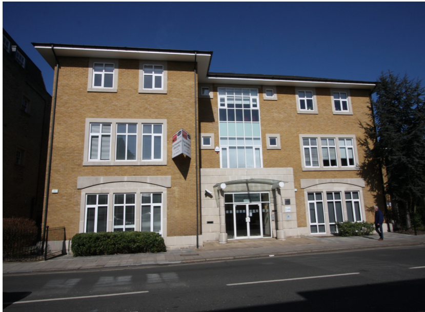
Tall 3 storey office development
