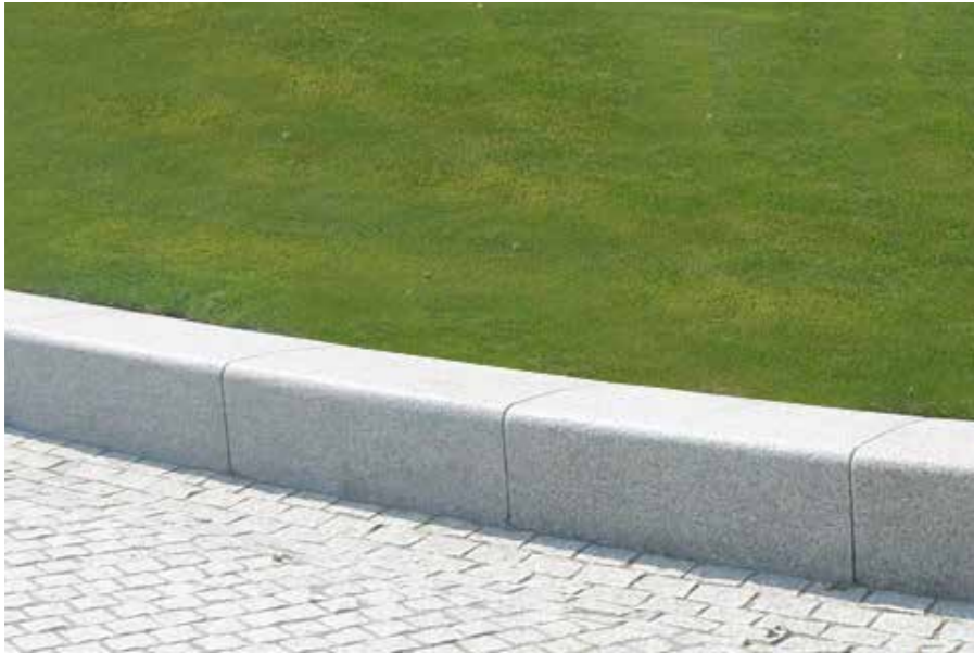
Granite seating edge with lawn to inner courtyard
