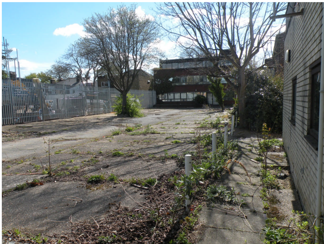
Plate 2. View of the site looking south east.
