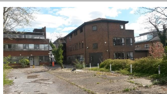
FIGURE 6: REAR VIEW OF EXISTING BUILDINGS
