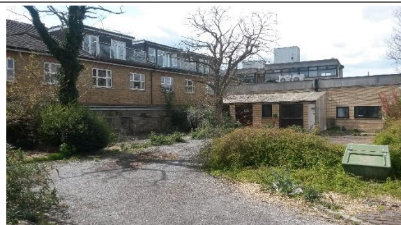
FIGURE 5: EXISTING BUILDING AT SOUTH-WEST PART OF THE SITE
