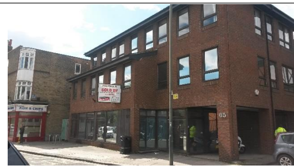
FIGURE 4: FRONT VIEW OF EXISTING BUILDING
