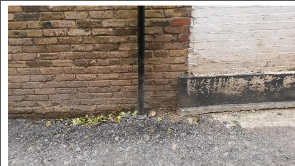
FIGURE 9: RAINWATER PIPE AT THE SITE
