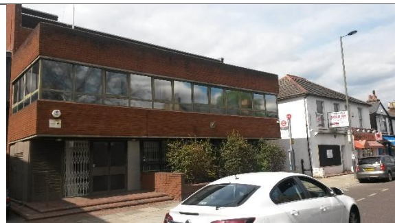
FIGURE 3: FRONT VIEW OF EXISTING BUILDING
