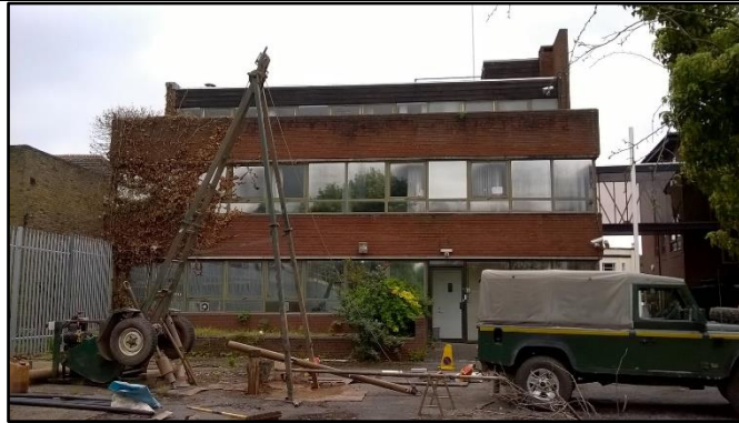
Photo 4 – Building B1 (northern)
