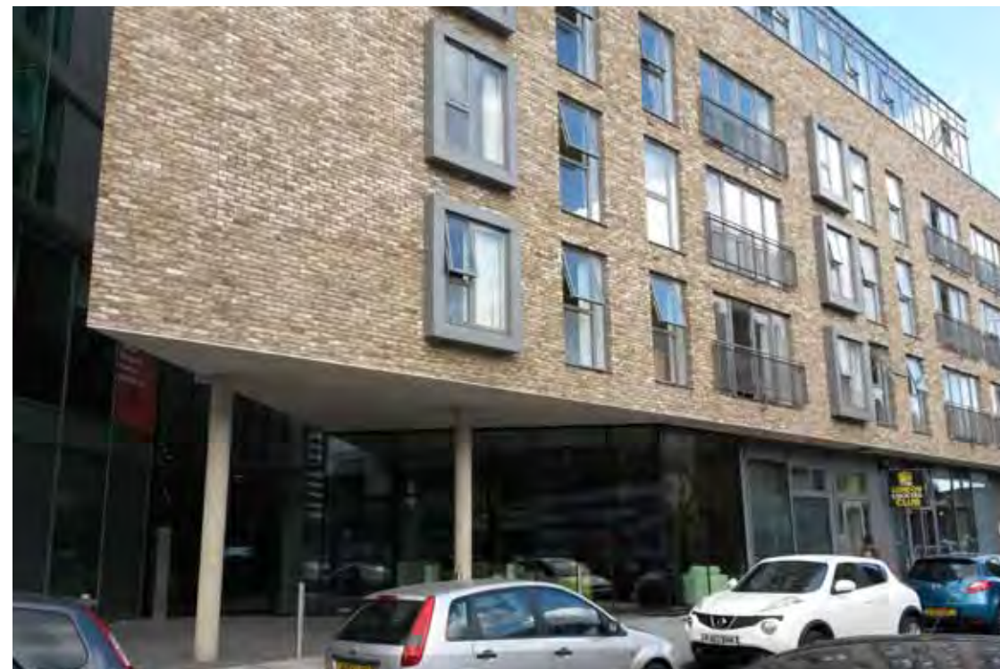
Brick upper storey facade projects over set back ground floor, forming natural canopy
