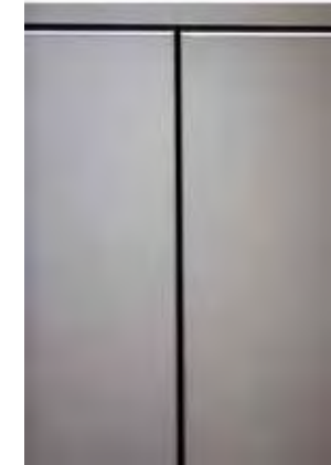
Top floor elements expressed in metal panel finish
