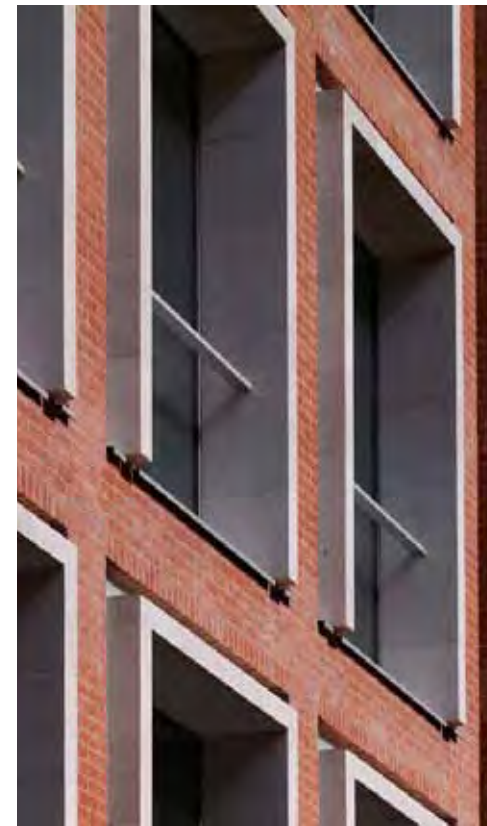
Feature surround recon stone elements to windows set in deep brick reveals
