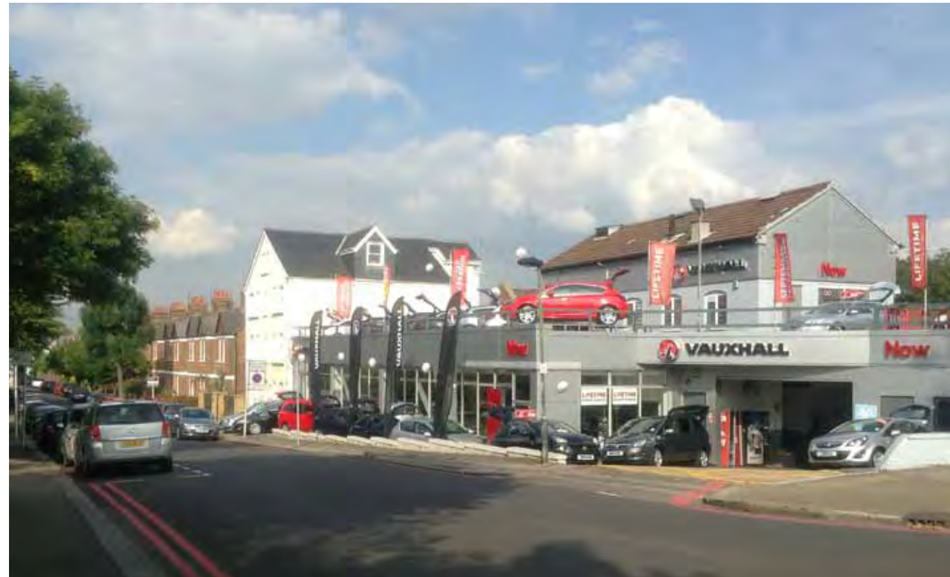
5 North Road corner: car dealer with three / four storey elements
