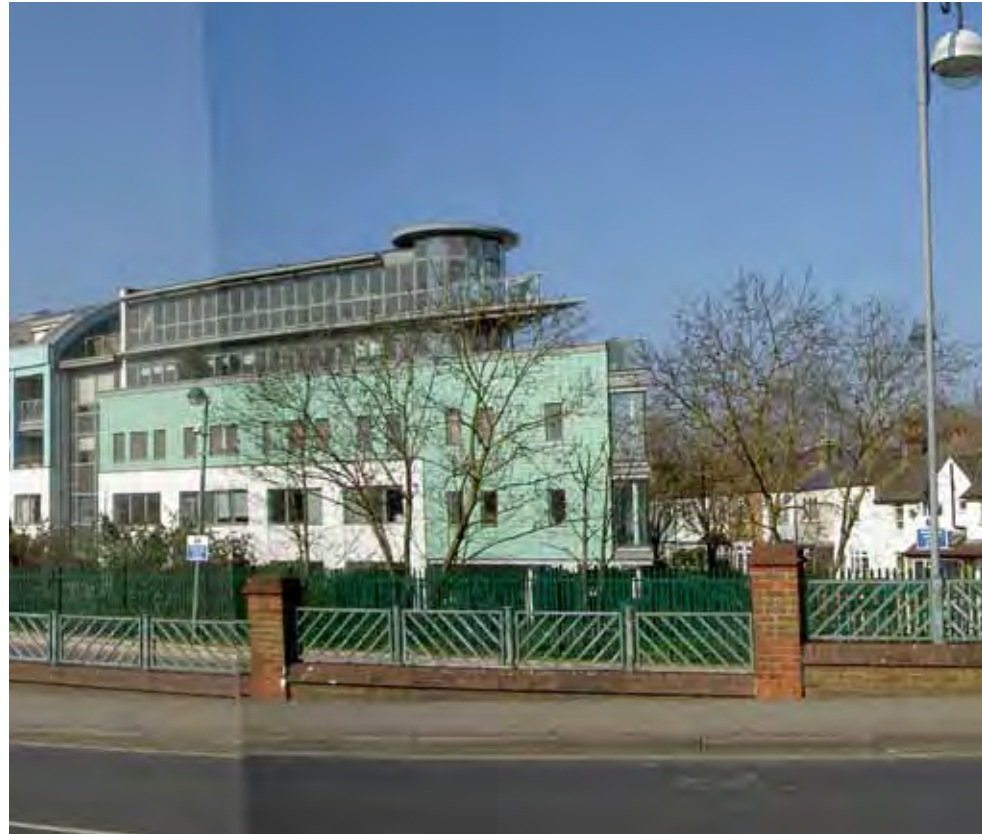
1 Falstaff House from Manor Road - recent mixed use development
