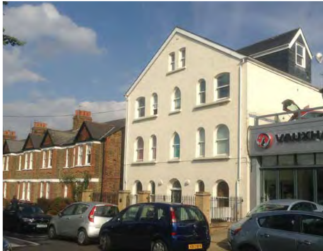
4 North Road four-storey abuts residential terraces
