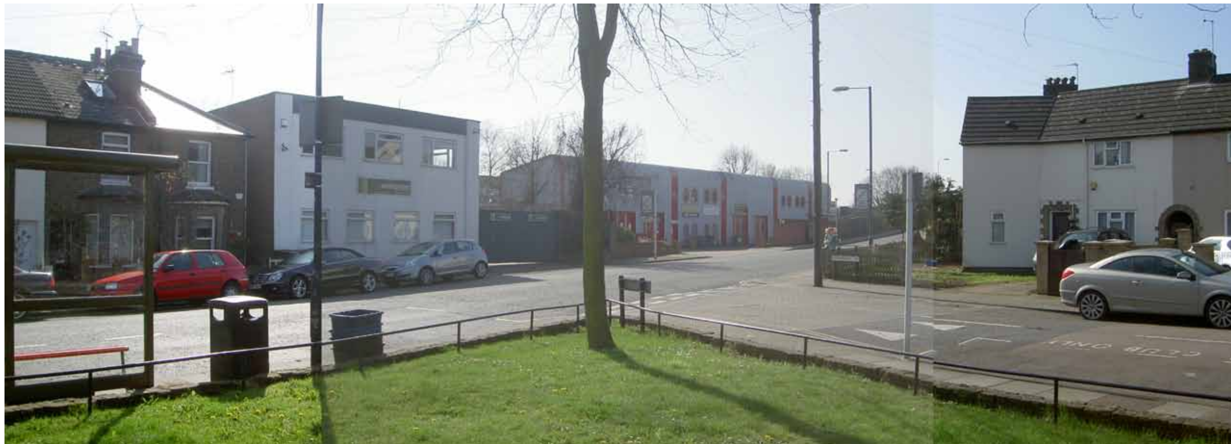
2 View of site looking south from Gainsborough Road junction showing Car Club space in right foreground
