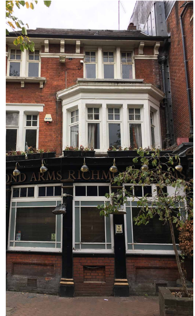
Picture 11 West Elevation
