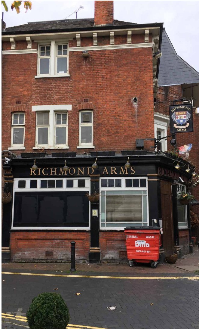
Picture 9 North Elevation
