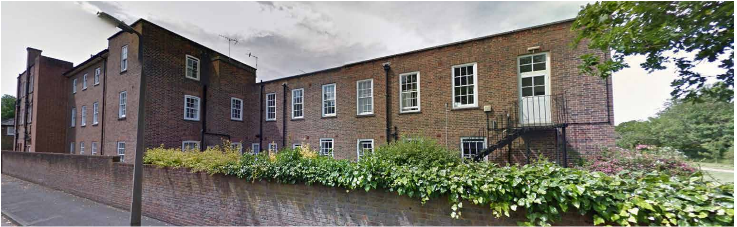
View of east wing from Martingales Close
