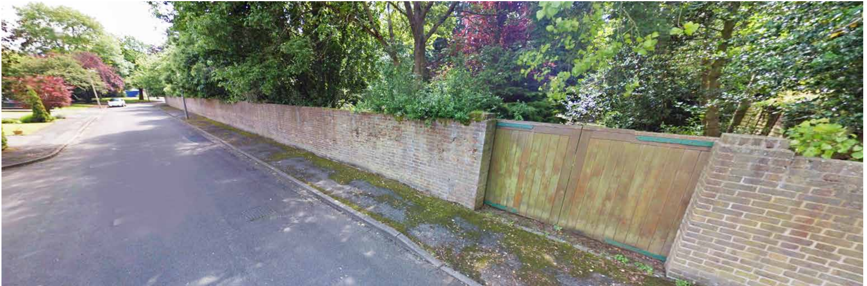
View of rear access to site from Martingales Close
