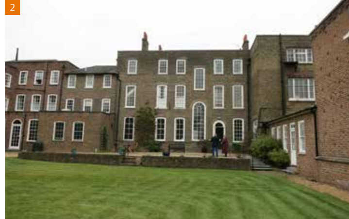
Listed building on site, North side
