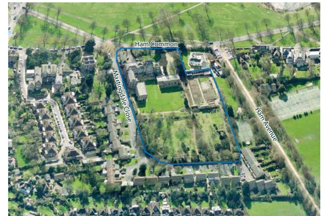
Aerial view of site looking south
