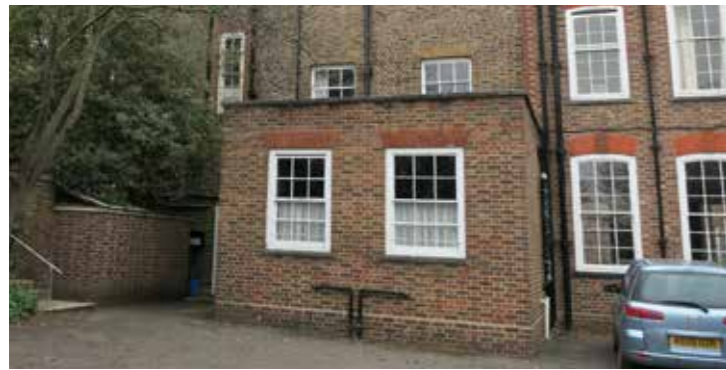
Front elevation later addition
