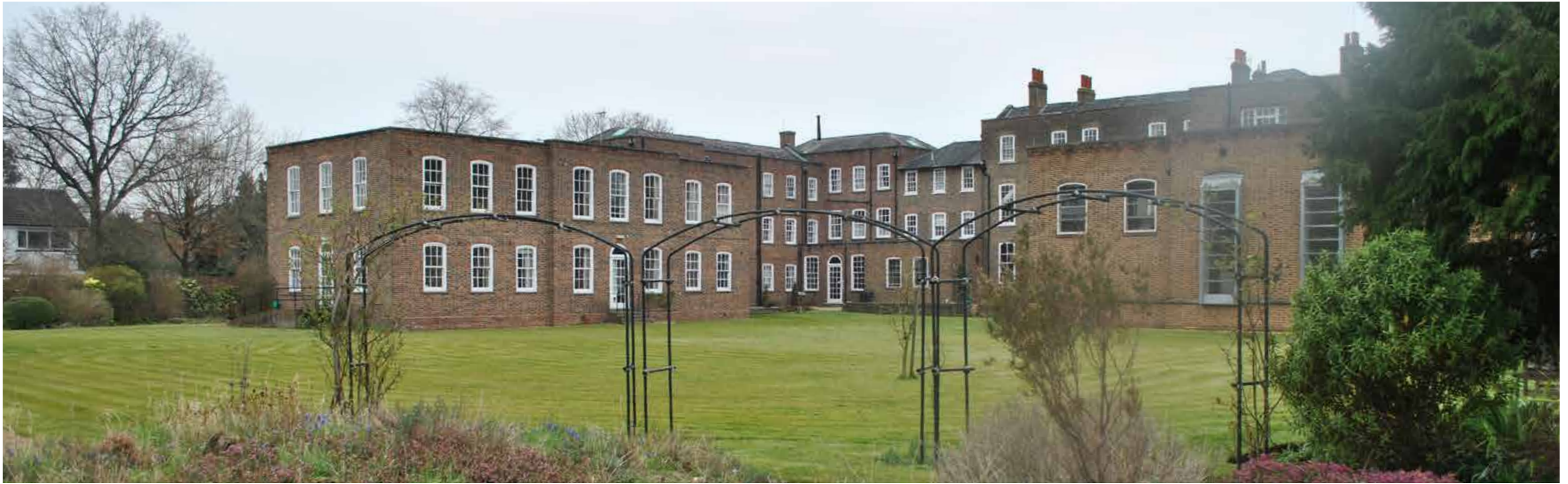
View of rear elevation
