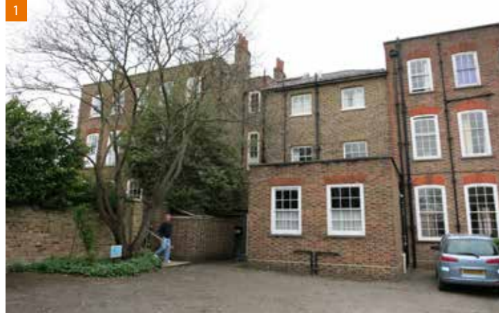
Listed building on site, South side
