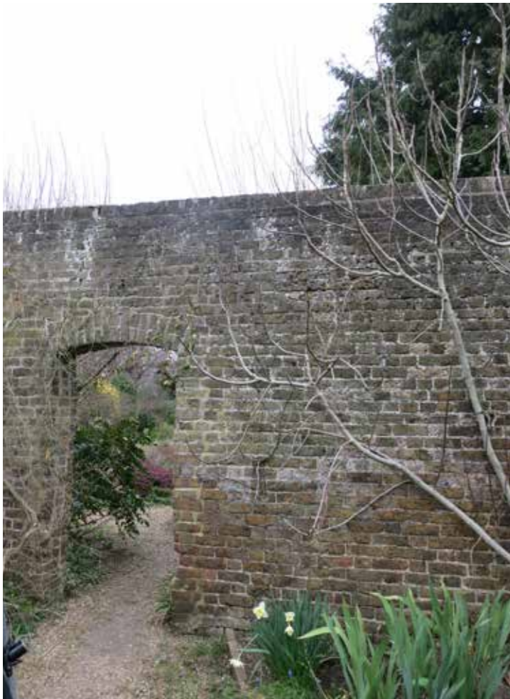
View of walled garden entrance
