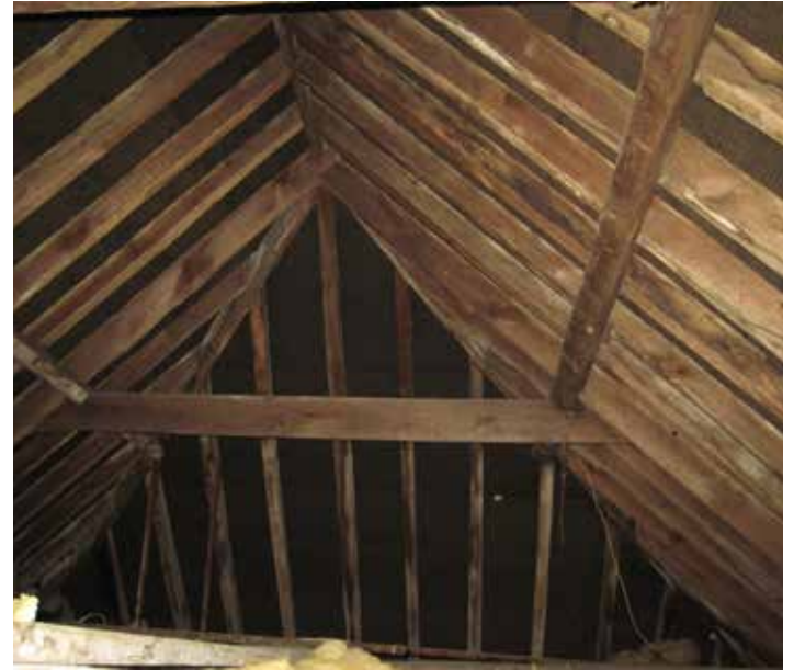
View inside roof hatch
