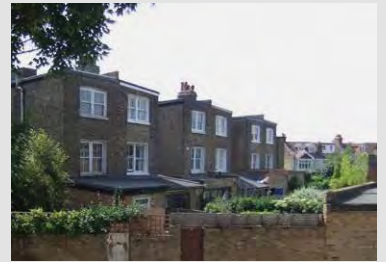
Rear of Elm Grove Road properties
