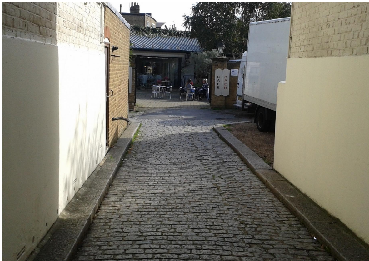
GRANITE SETTS TO CARRIAGEWAY
