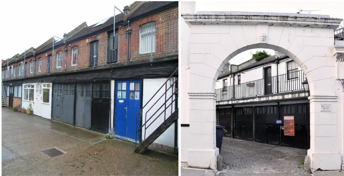
LEFT - MEWS GARAGES OFF BRACKNELL GARDENS
