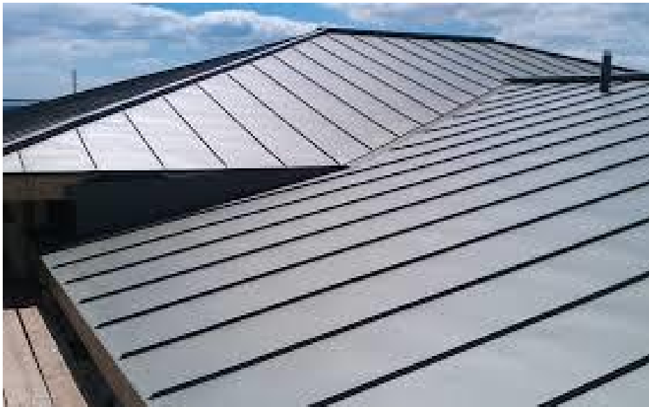
ZINC ROOFING WITH STANDING SEAMS
