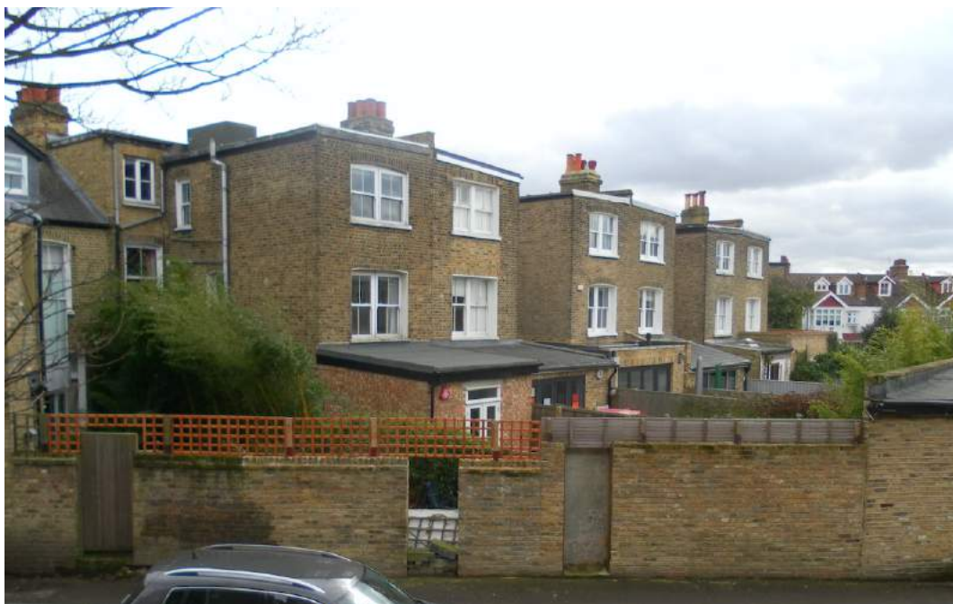
Figure 5.3 – Nos. 4-14 Elm Grove Road (Rear Elevations) and Aerial Photograph
