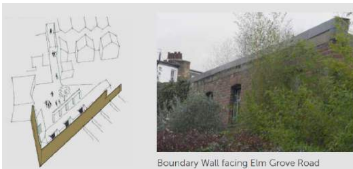
Figure 2.2 – Stable Wall of Site (approx. 4.5m high)
