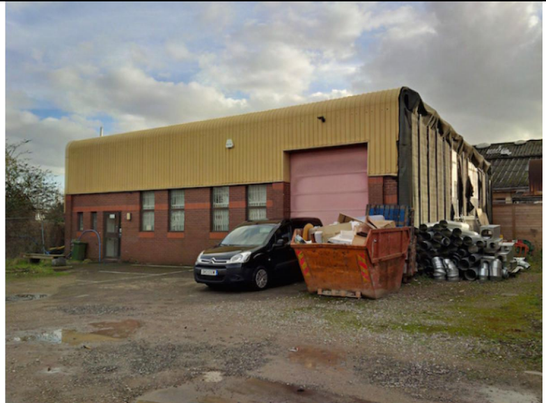
Photo 1: Current warehouse (built structure) on site.
