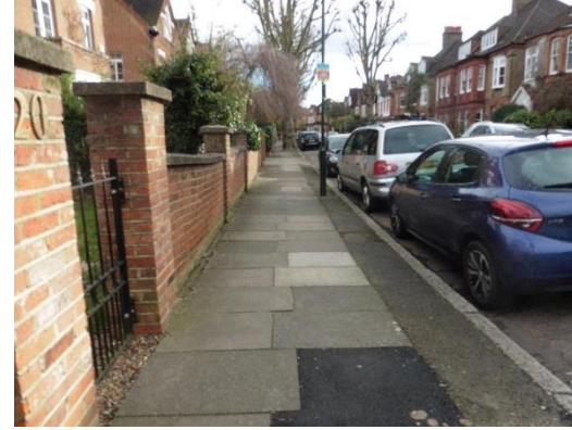
Link 19 – Radnor Road (Western footway)
