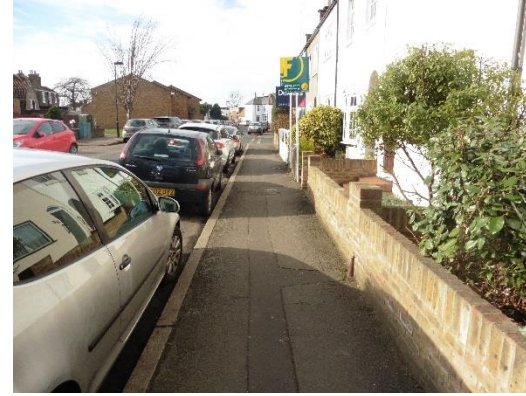
Link 3 – Edwin Road (Northern footway)
