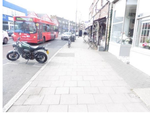
Link 18 – Heath Road (Northern footway)
