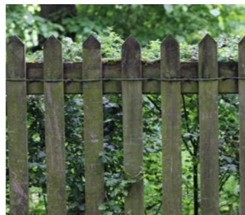
Palisade fencing around Woodland Quarters
