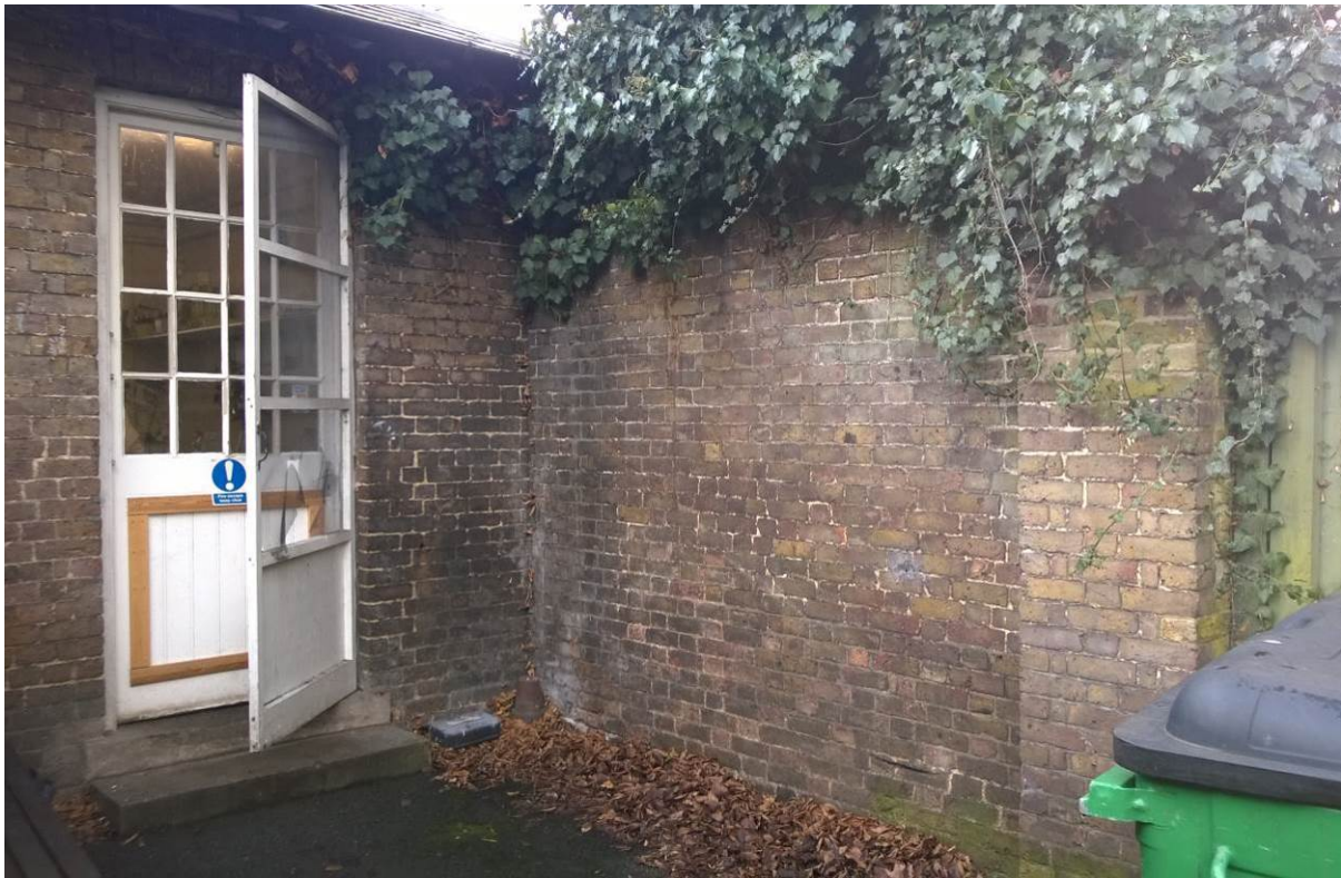
Photograph 25 – South end cross wall at junction of stables building.
