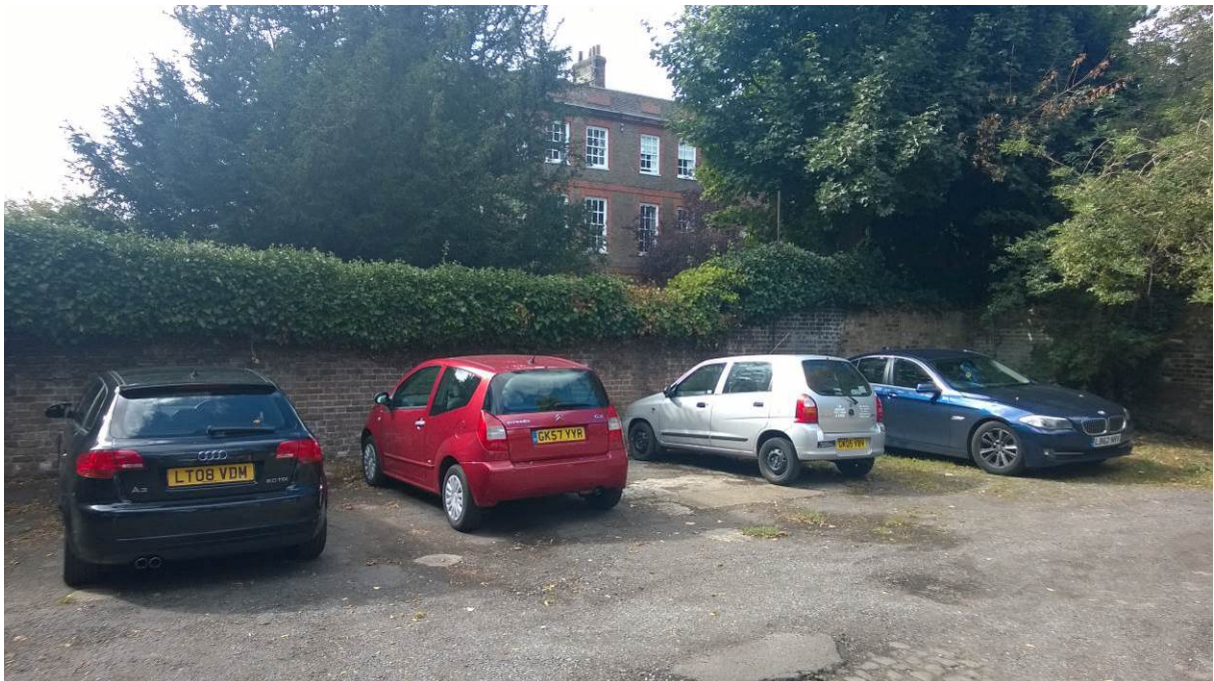
Photograph 2 – North end of boundary wall.
