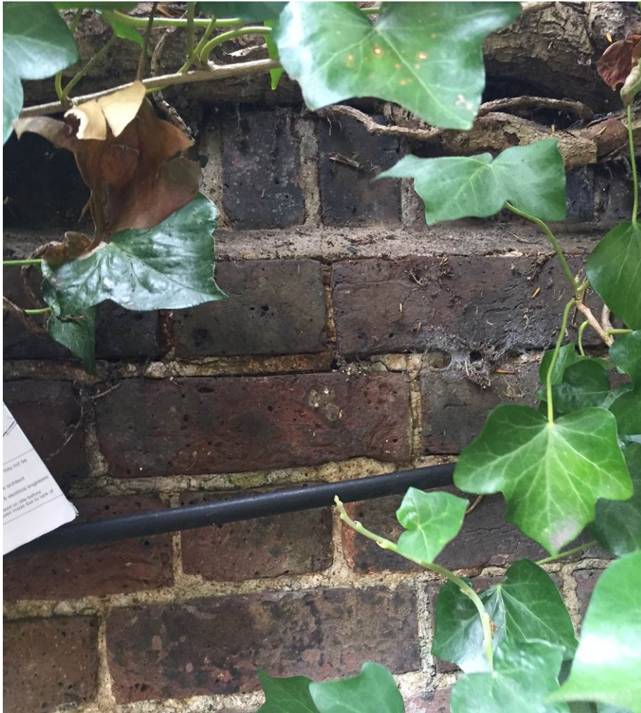
Photograph 11 – Cementitious mortar pointing to top of the wall.
