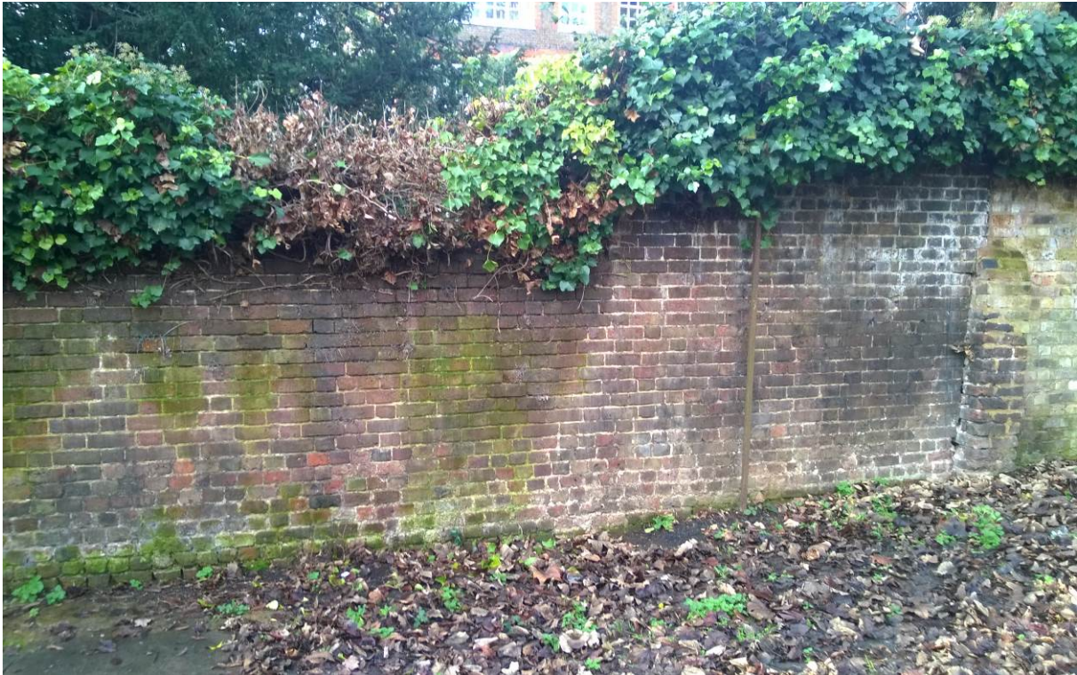
Photograph 13 – North end of wall, change in wall height.
