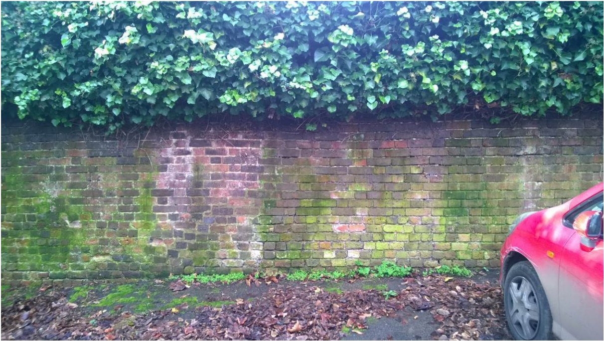
Photograph 5 – Near south end, area of rebuilding to wall.
