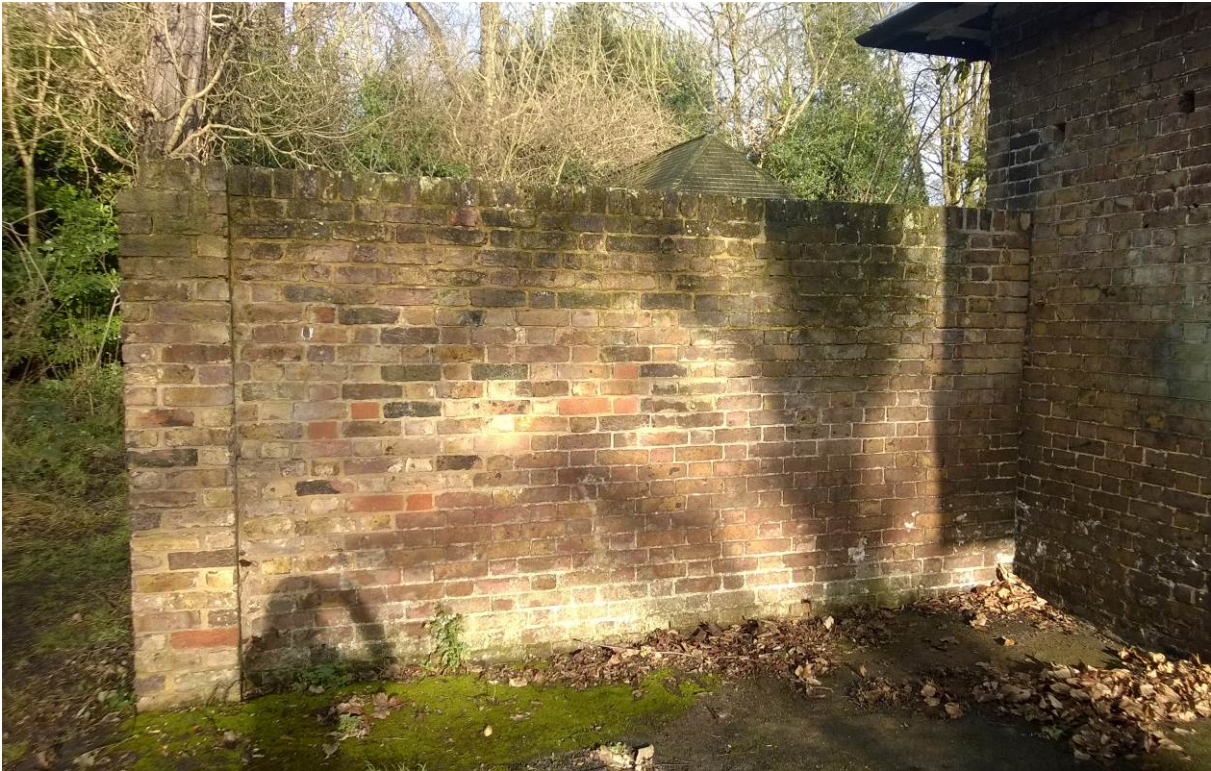
Photograph 19 – Continuation of north wall and junction with stables building.
