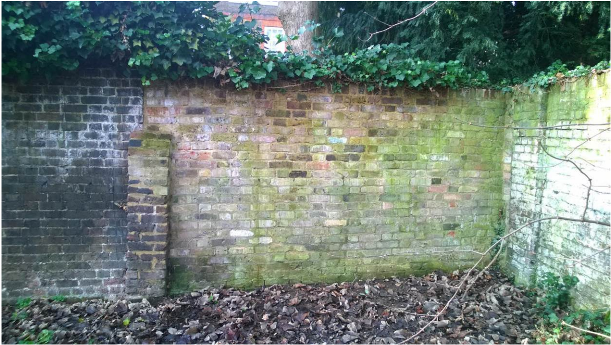
Photograph 15 – Junction of north end of wall and North cross wall, change in construction at pier- wall is likely rebuilt because of proximity of large trees to west elevation.
