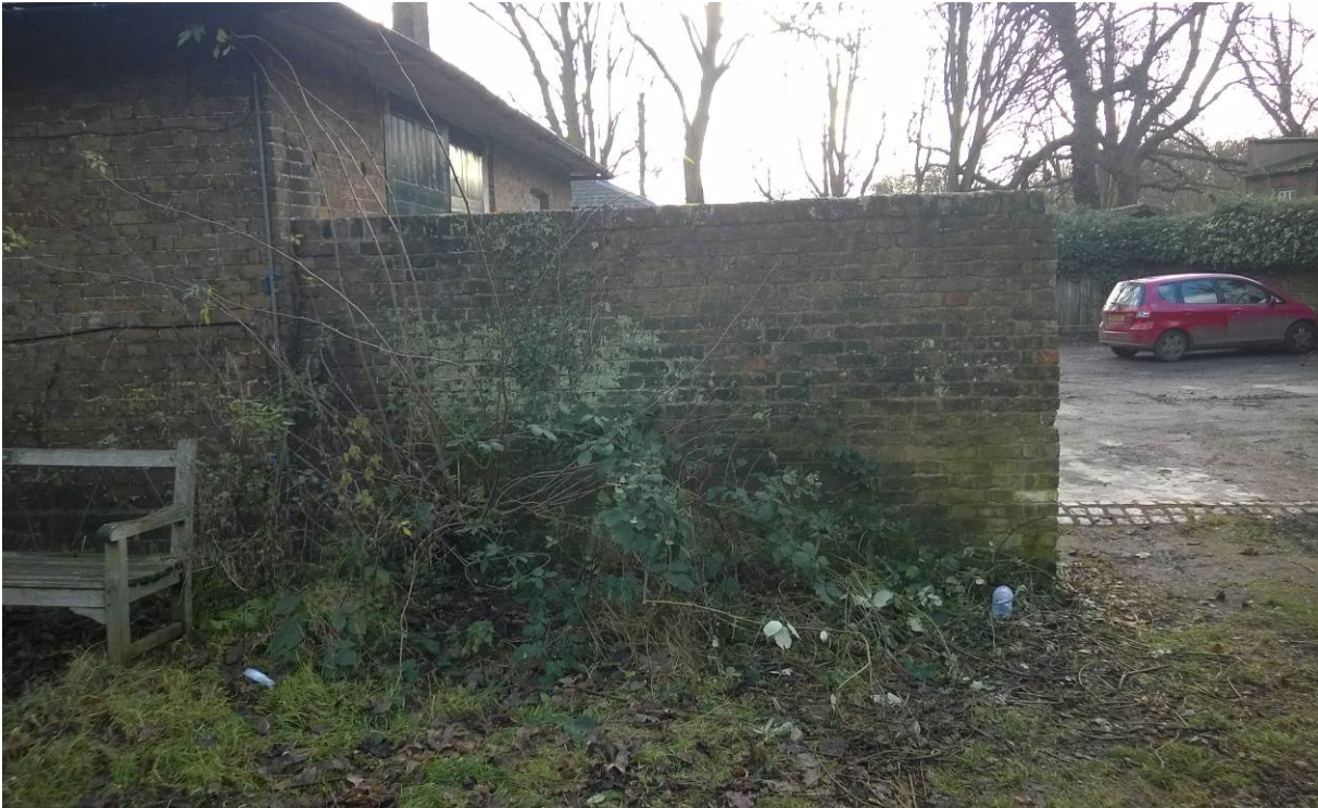
Photograph 21 – Vegetation growth in close proximity to North elevation of north end cross wall.
