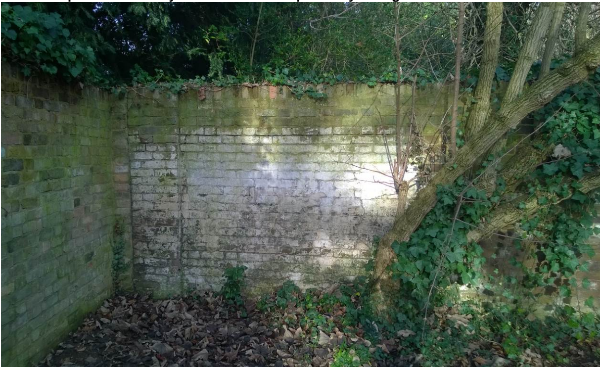
Photograph 15 – Junction of north end of wall and North cross wall, change in construction at pier- wall is likely rebuilt because of proximity of large trees to west elevation.
