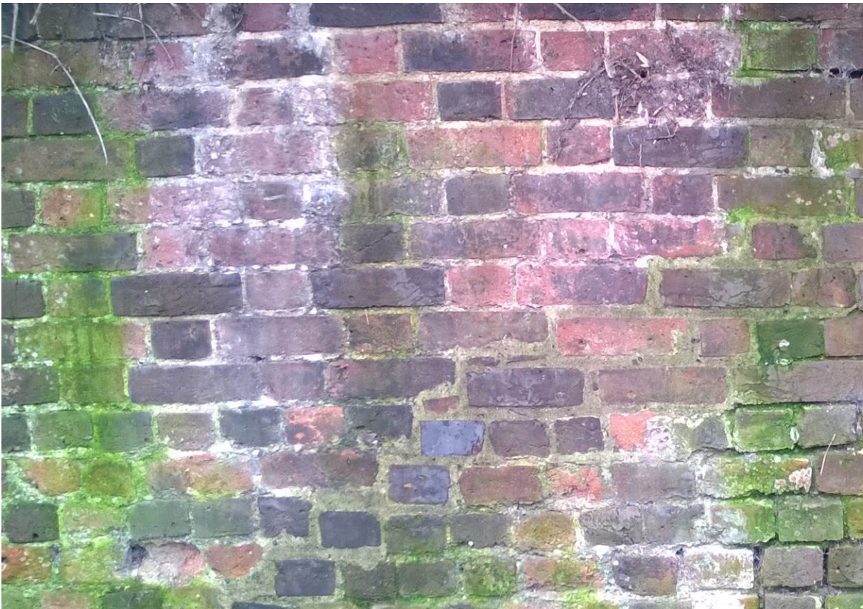
Photograph 6 – Cementitious mortar to rebuilt area of wall.
