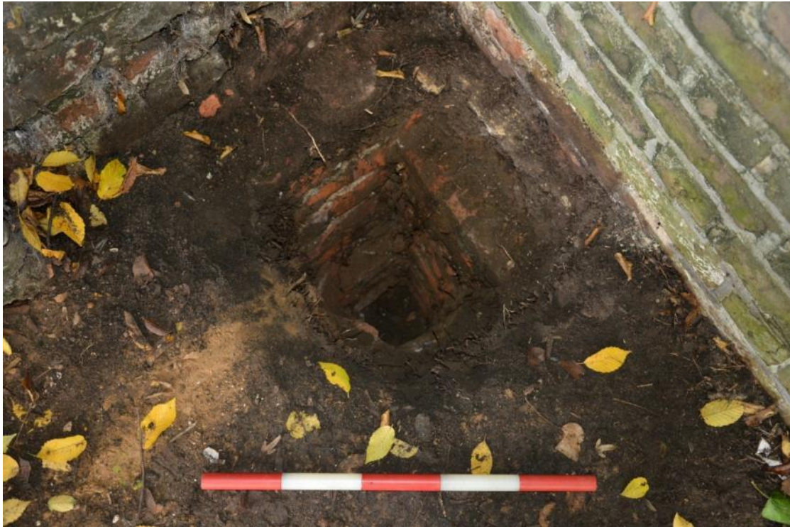
Figure 16: TP4 - exposed footings of two phases of construction. Facing W. Scale 0.5m.
