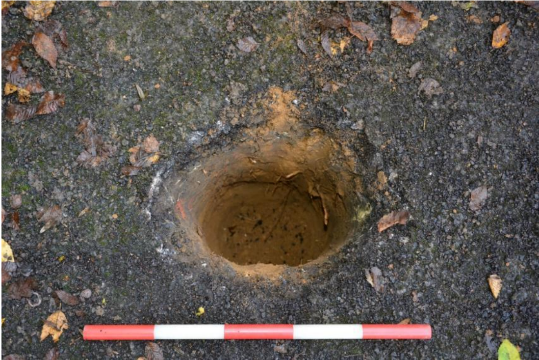
Figure 21: Borehole 2 prior to window sampling. Scale 0.5m.
