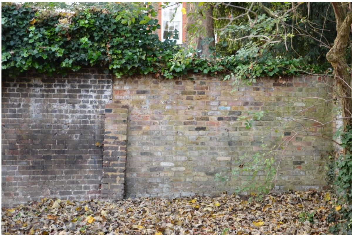
Plate 6 Northern end of the long western yard wall with later blocking. Viewed from the east.
