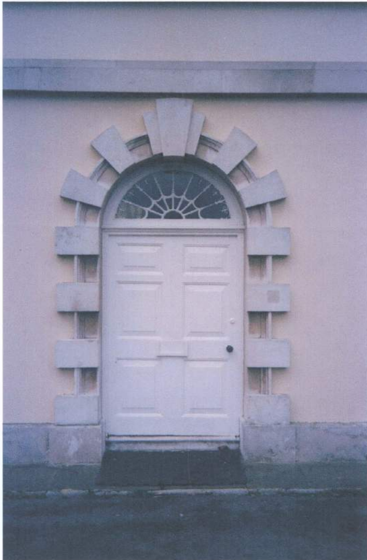
Figure 18). Exterior South façade, main entrance door
