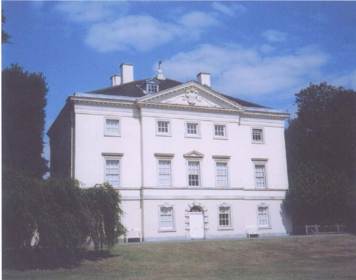
Figure 1). External view of Marble Hill House, South elevation, February 2004
