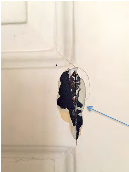
Figure 11: Door to Hall
