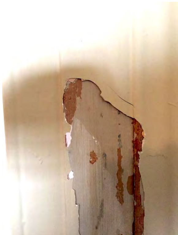
Figure 21: South west door, architrave
