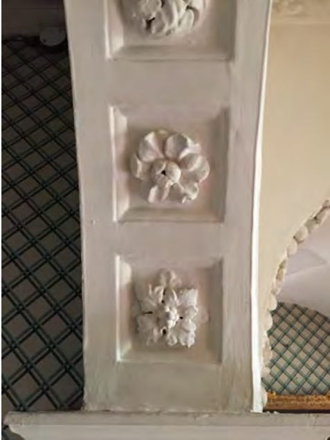
Figure 7: Screen intrados raised detail
