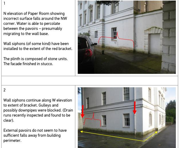
Small trench installed at wall perimeter (yellow arrow) – filled with pea gravel – which was very wet.
