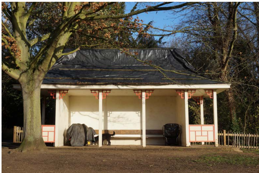
Fig 46 Today the shelter is without its copper roof which was stolen some years ago
