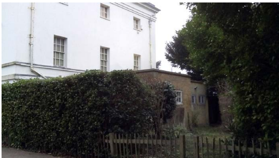
Fig 56 The toilet block built in 1909
