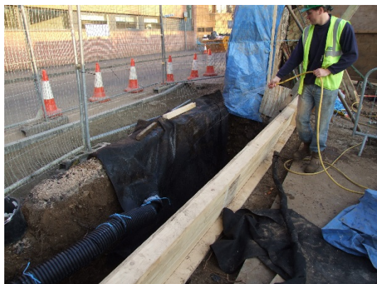
Photograph 4: Trench sides protected from drying by wet Hessian
