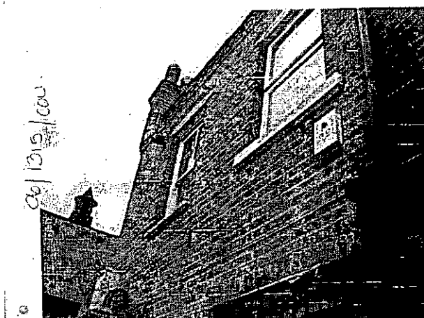
Figure 1 – rear facing first floor window of the upper floor flat to 277 Sandycombe Road with existing building in the background
