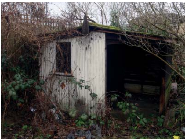
Plate 5. Timber and corrugated asbestos sheet shed with concrete floor.
