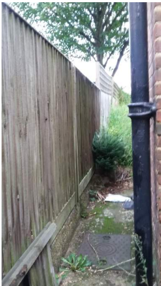
Plate 5 View along western access to rear garden, facing northeast
