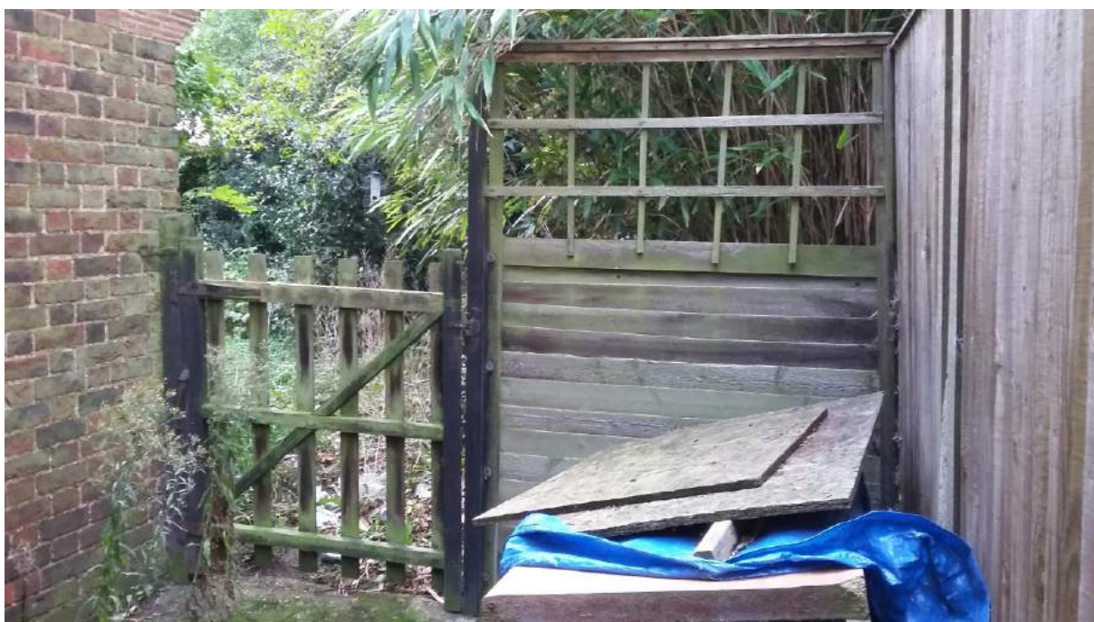
Plate 4 View of gated entrance to rear garden of The Firs, facing southwest
