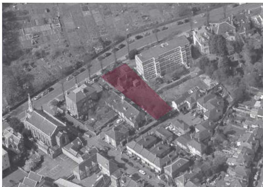
Figure 2 Bird's eye view of existing Building
