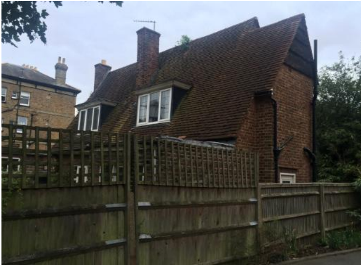
Appearance from grounds of Heron House
