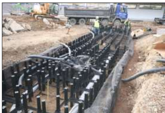
Soil cell image 1: The individual Silva Cells can be assembled in layers and service ducting threaded through before filling with soil and fitting the reinforced tops.
