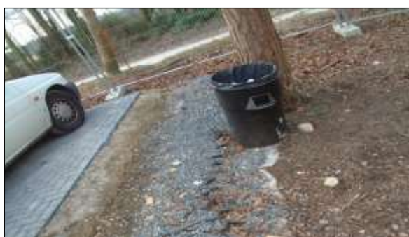
New surfacing image 4: A conventional concrete haunching can be used to retain new surfacing as long as it is not dug into a trench - here it is placed on top of the CellWeb layer.
