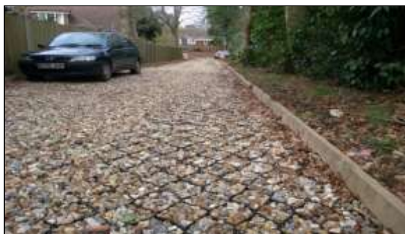
New surfacing image 6: Wooden board pinned in place or held in position with backfilled topsoil can provide more informal and rustic surface edging.
