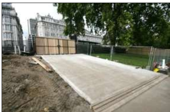
New surfacing image 8: This temporary access for heavy construction traffic on the outer edge of a RPA is a concrete slab cast above ground level and will be removed when the project is completed.
