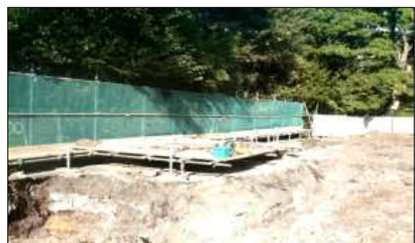
Ground protection image 4: A scaffold framework attached to the main scaffold fencing can be used to support either scaffold planks or plywood to create an elevated platform with a gap beneath.
