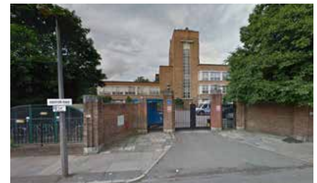
Access Point 5 - Egerton Road near Craneford Way
