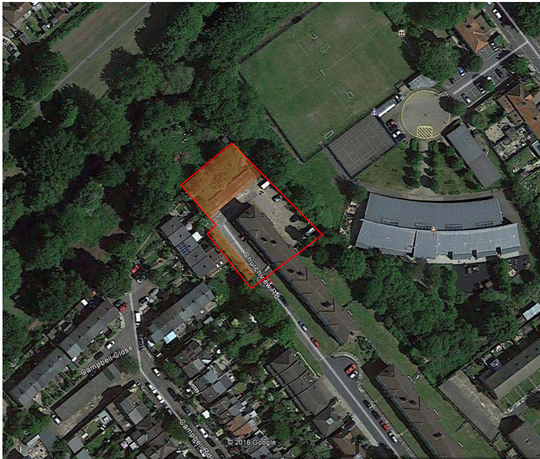
Figure 2 - Aerial View of Development Site. Proposed development area outlined in red. Shaded area indicates area relevant for drainage strategy.
