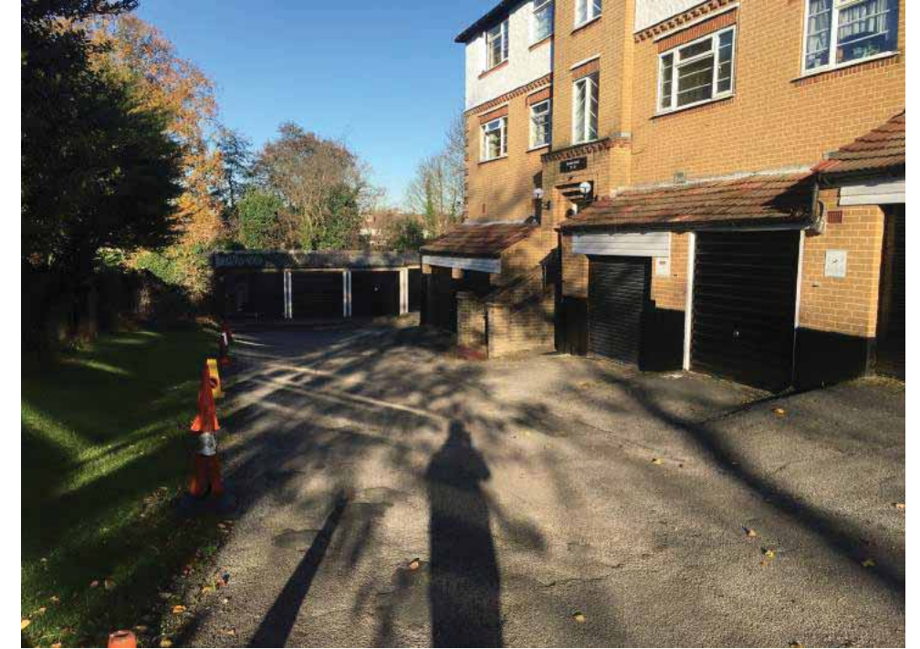
FIG. 13 VIEW 3 EXISTING GARAGE LOOKING NORTH WITH NO.72-75 IN FOREGROUND
