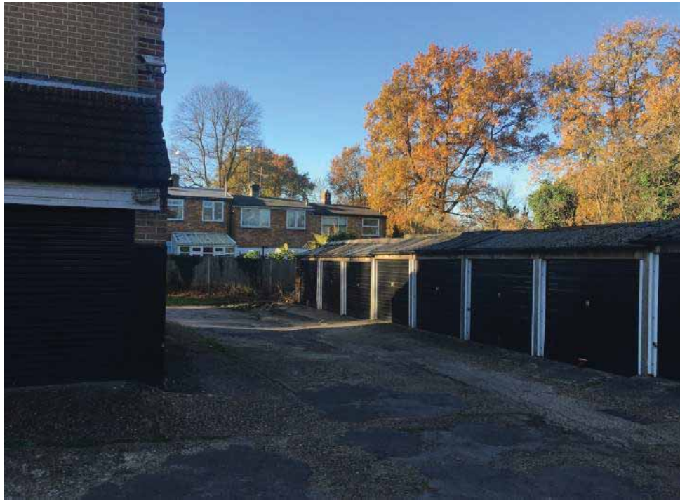
FIG. 27 VIEW 6 EXISTING GARAGE LOOKING NORTH WEST WITH NO. 17-20 CAMPBELL CLOSE IN BACKGROUND
