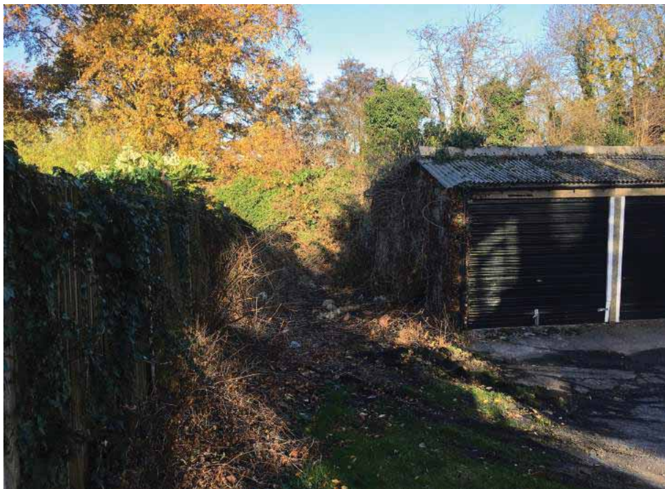
FIG. 14 VIEW 4 EXISTING GARAGE LOOKING NORTHWEST
