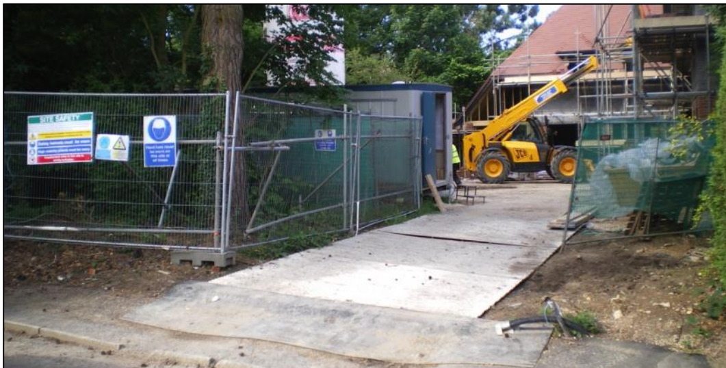
Vehicular ground protection trackway
