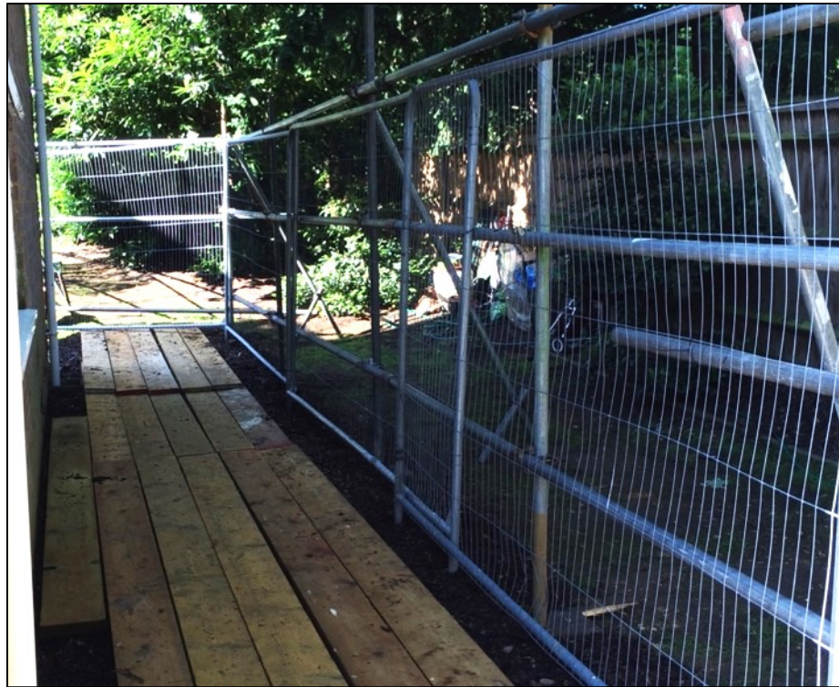
Scaffold board pedestrian ground protection
