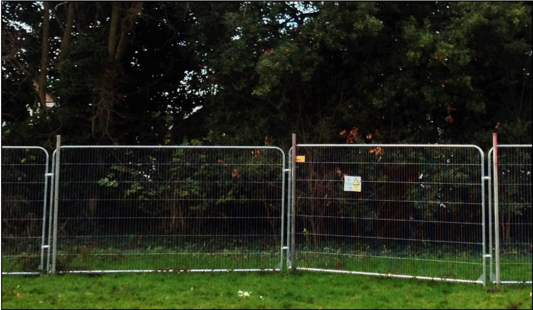
Weld-mesh panels on scaffold uprights
