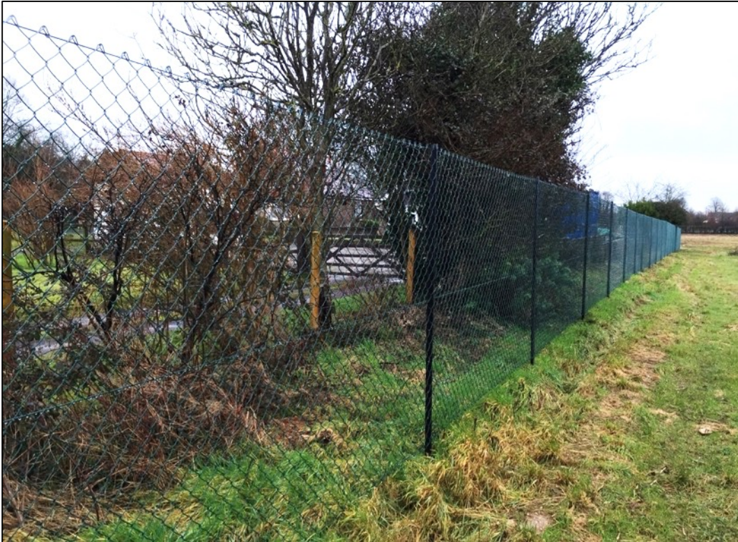
Chain-link on angle-iron uprights
