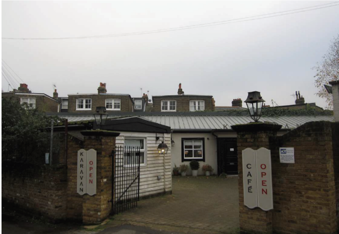
Existing View (Northern Elevation)
