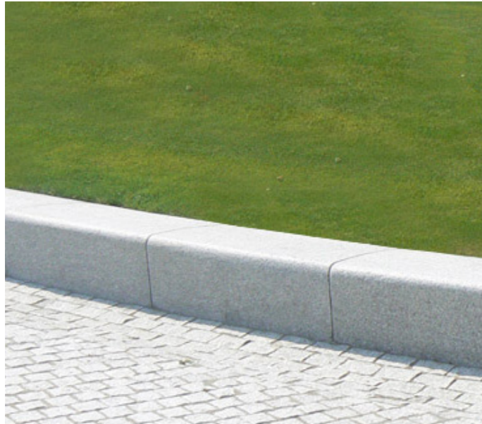
Granite seating edge with lawn to inner courtyard
