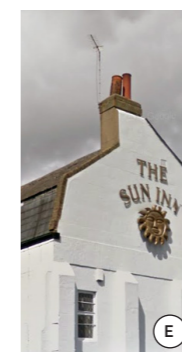
Irregular roof profile to neighbouring listed building
