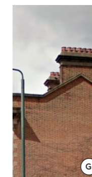
Irregular roof profile helps to emphasise traditionally detailed chimney stack
