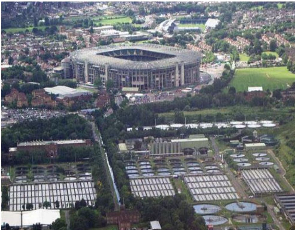
Aerial view of existing site from the north (Mogden Sewage Works in foreground)
