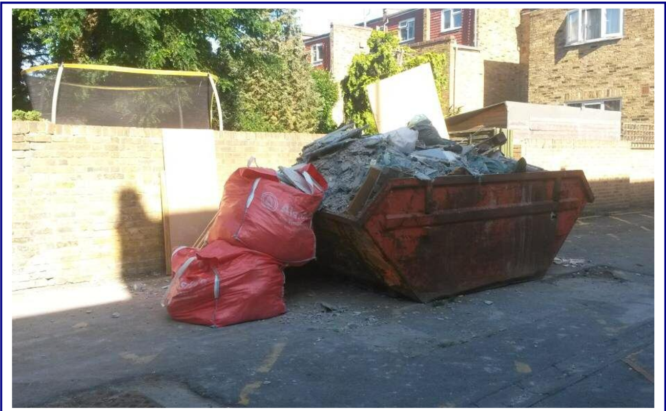
Photo 4: Skip located to the front of the onsite building.
