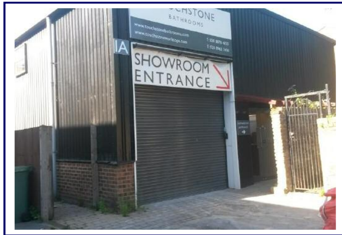
General view of the site. For further photos see Appendix B.
