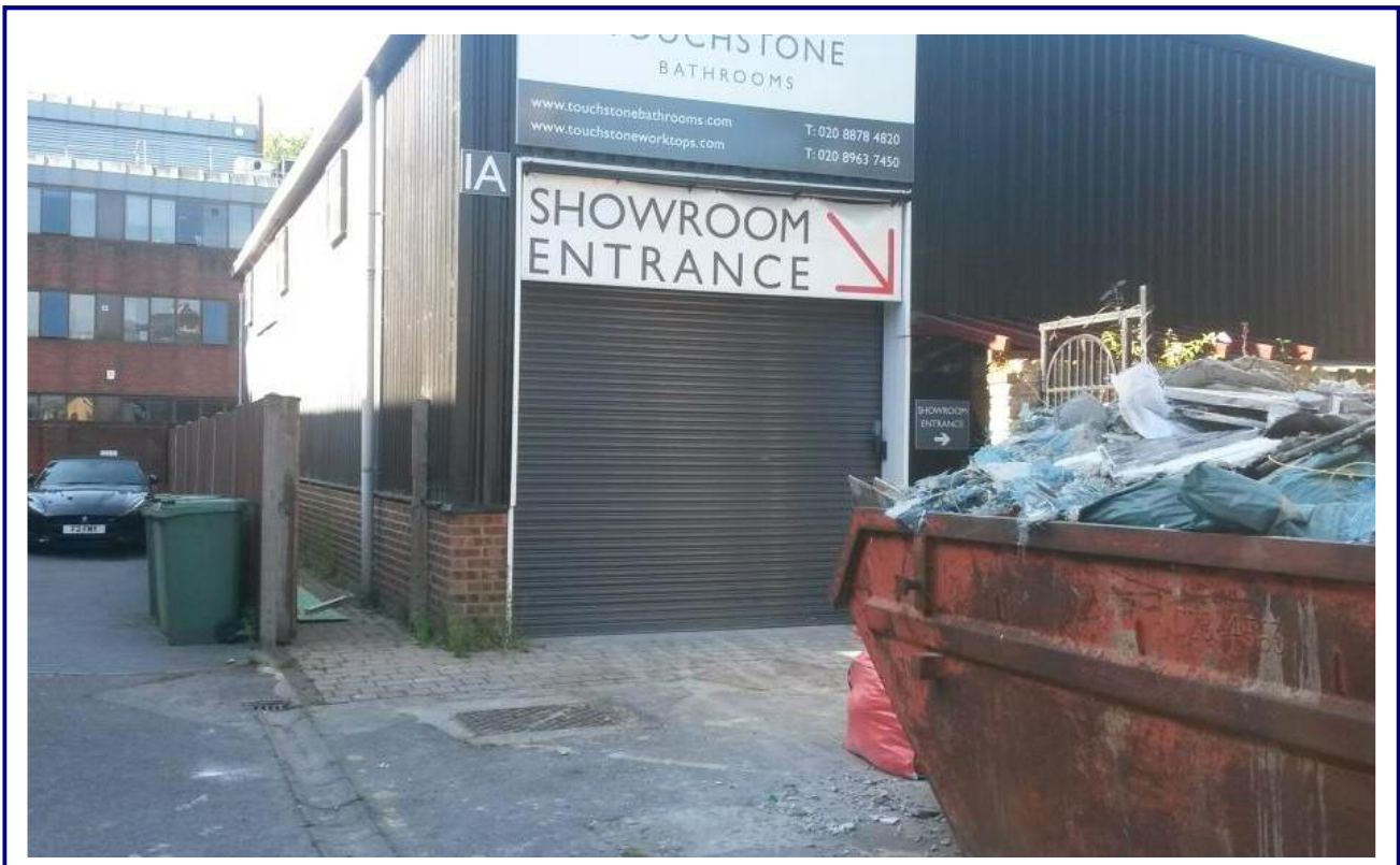
Photo 2: Front view of the site building with brick and metal cladding façade and external border.
